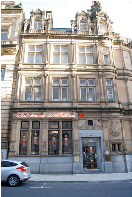
Photo showing main facade on Spring Gardens.
