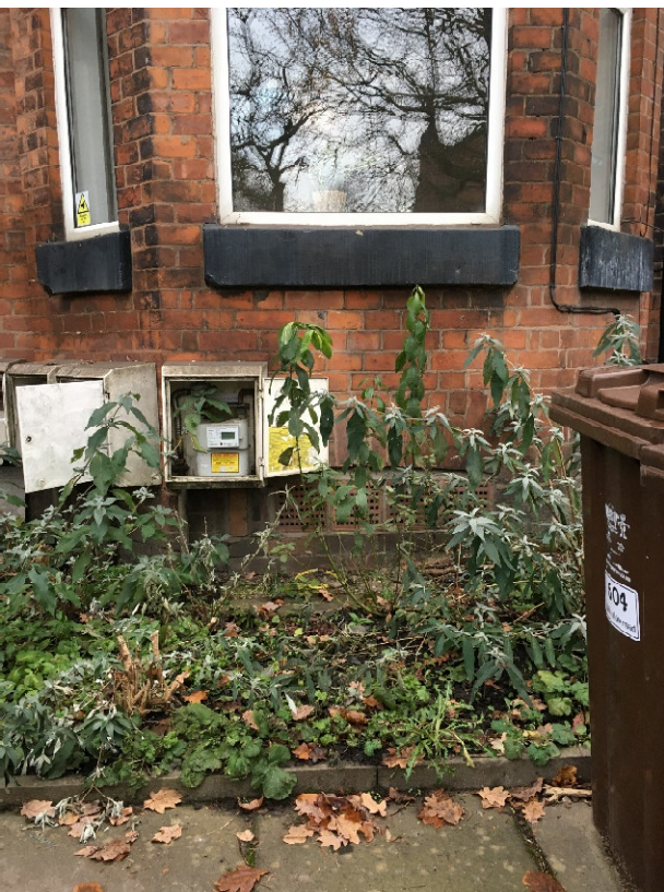
Figure 6.5. Existing basement front window
