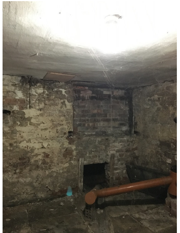
Figure 6.4. Existing basement rear window (internal view)
