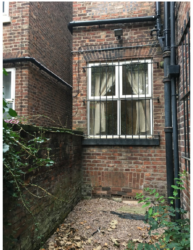
Figure 6.6. Existing basement rear window
