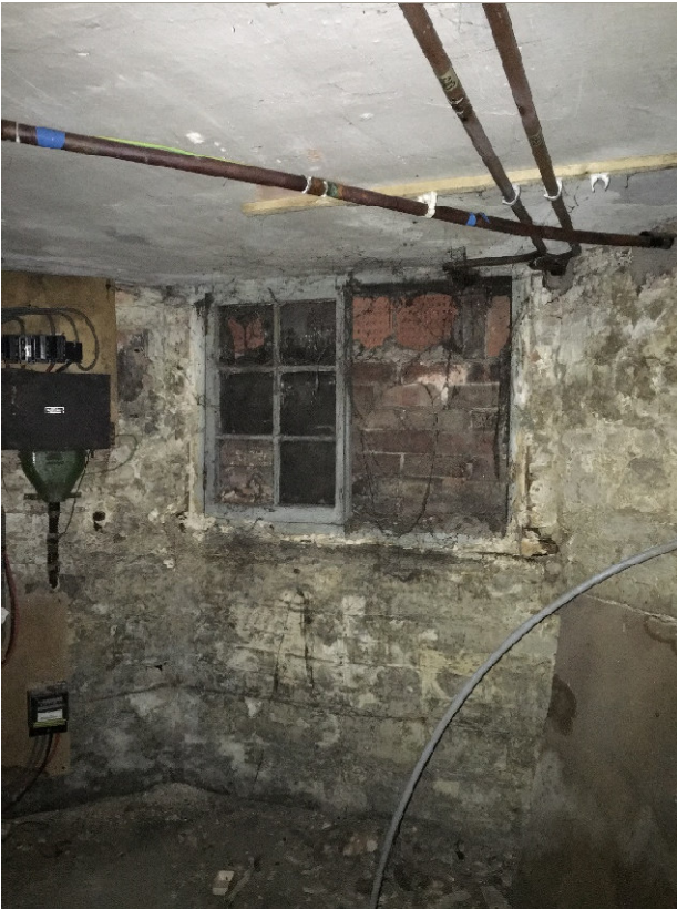
Figure 6.3. Existing basement front window (internal view)
