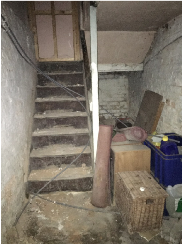
Figure 6.1. Existing internal stairs connecting ground floor apartment to basement, currently blocked up
