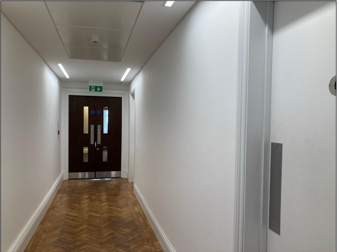
Original parquet flooring to eighth floor corridor
