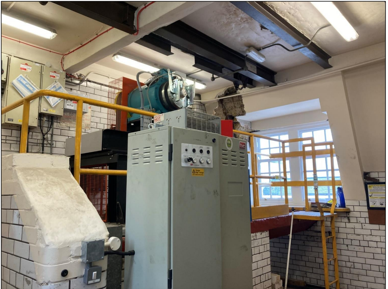
Lift motor room with original tiling
