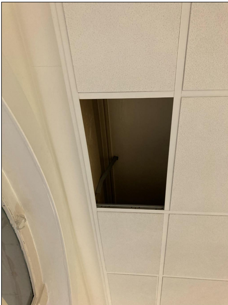
Original ceiling intact above modern suspended ceiling at first floor level
