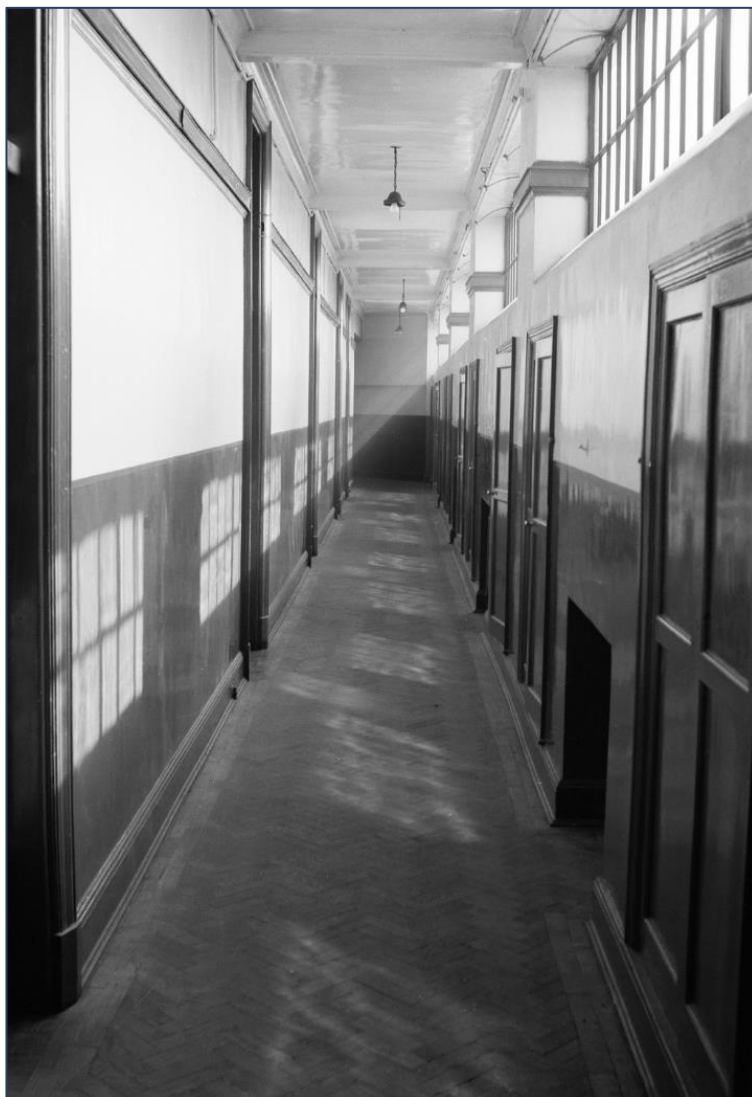
Figure 33 – Thirteenth floor corridor (1958)
