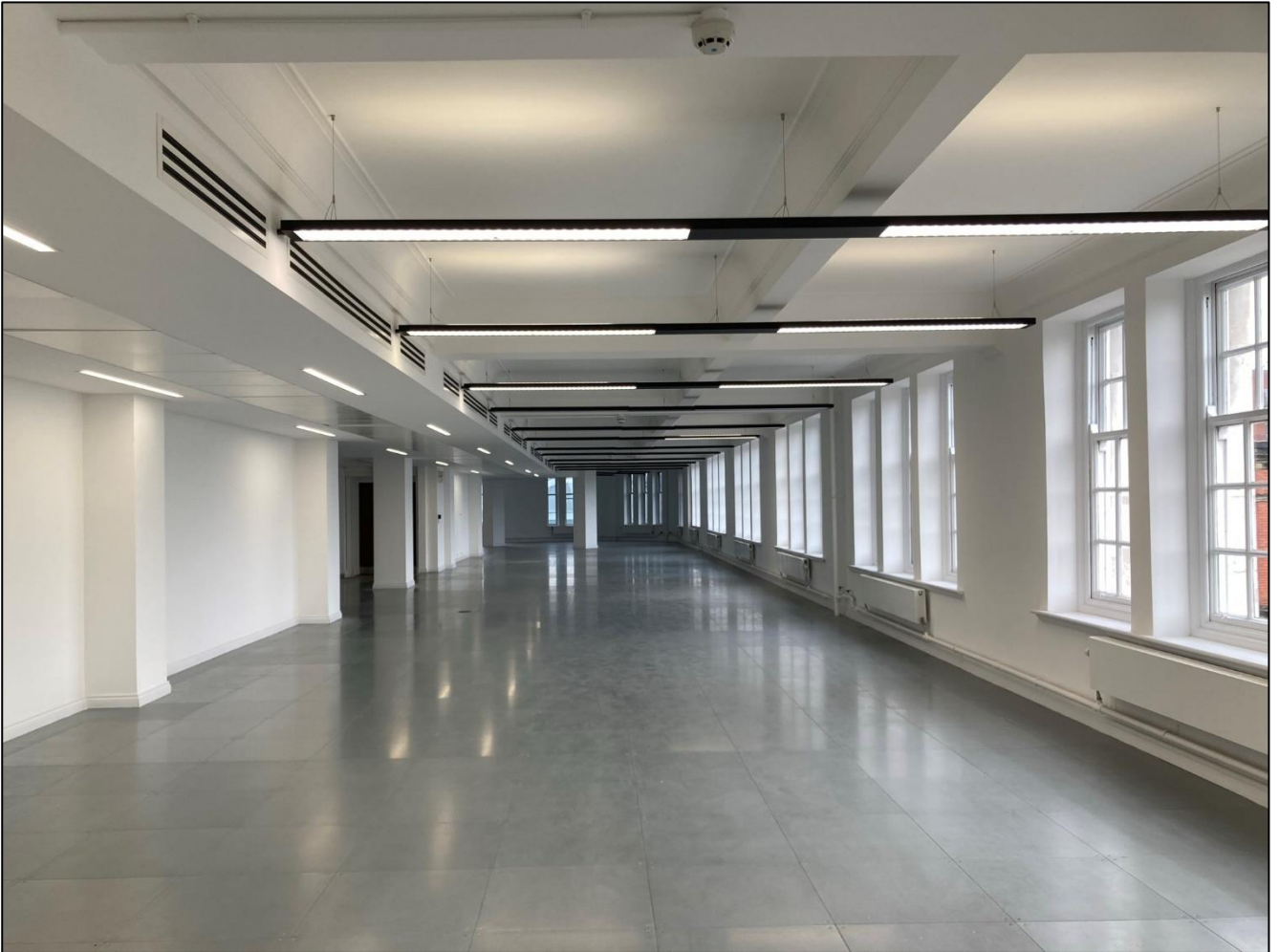
Raised floor on the eighth floor, with exposed original coved ceiling and non-original lights
