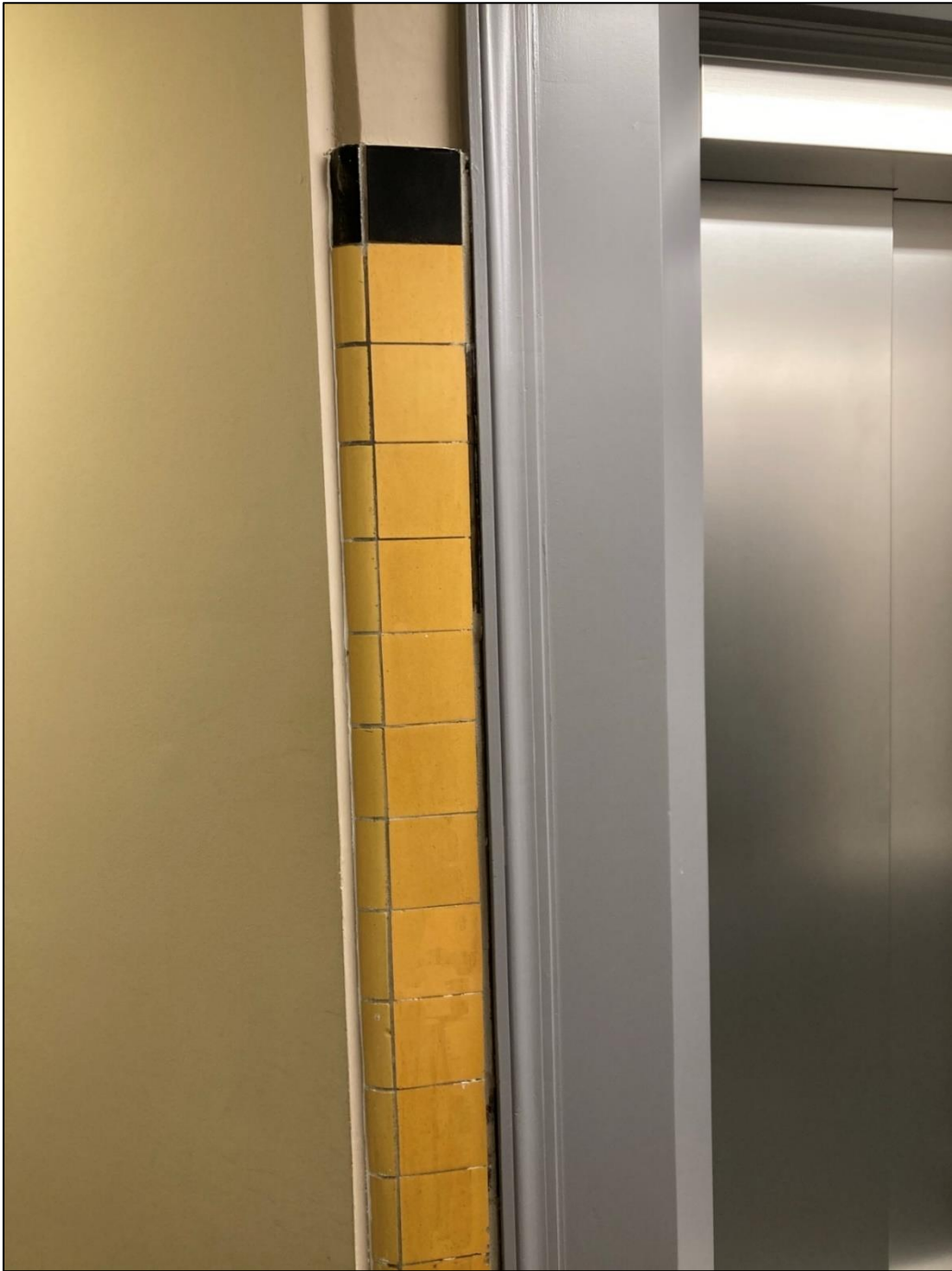
Original tiling adjacent to lift
