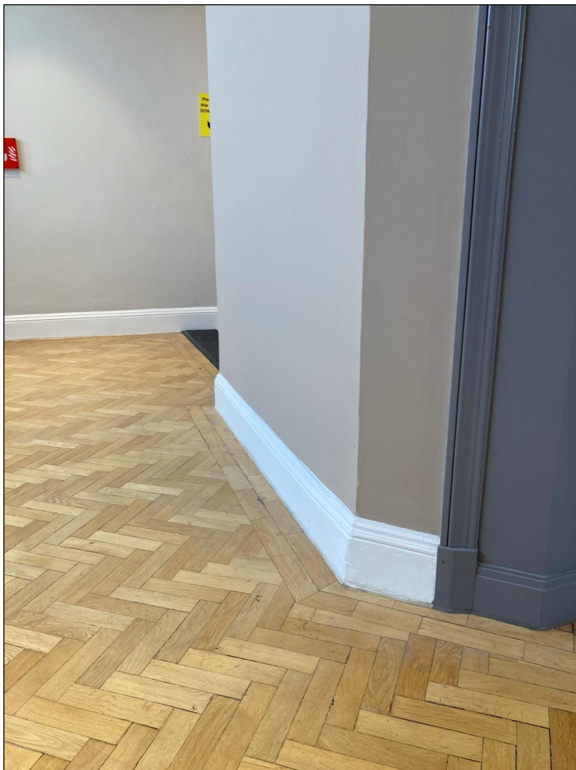
Original parquet flooring and skirting, thirteenth floor
