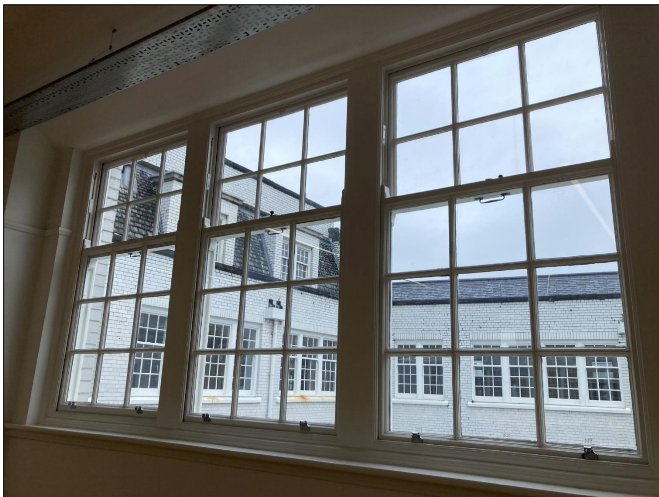
Thirteenth floor original windows
