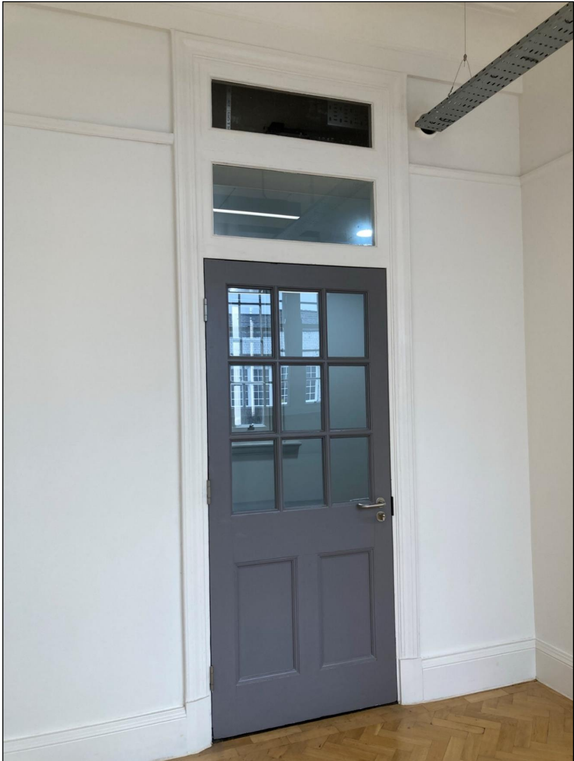
Example doorway on the thirteenth floor, door itself non-original.
