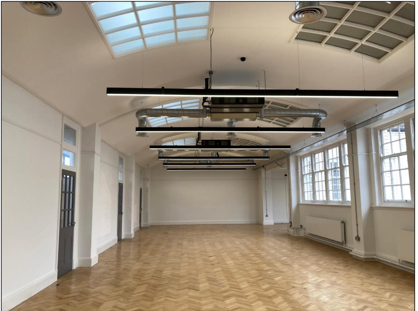
Original barrel ceiling with blocked up roof lights, thirteenth floor; wall nicks and doors denote original partitions
