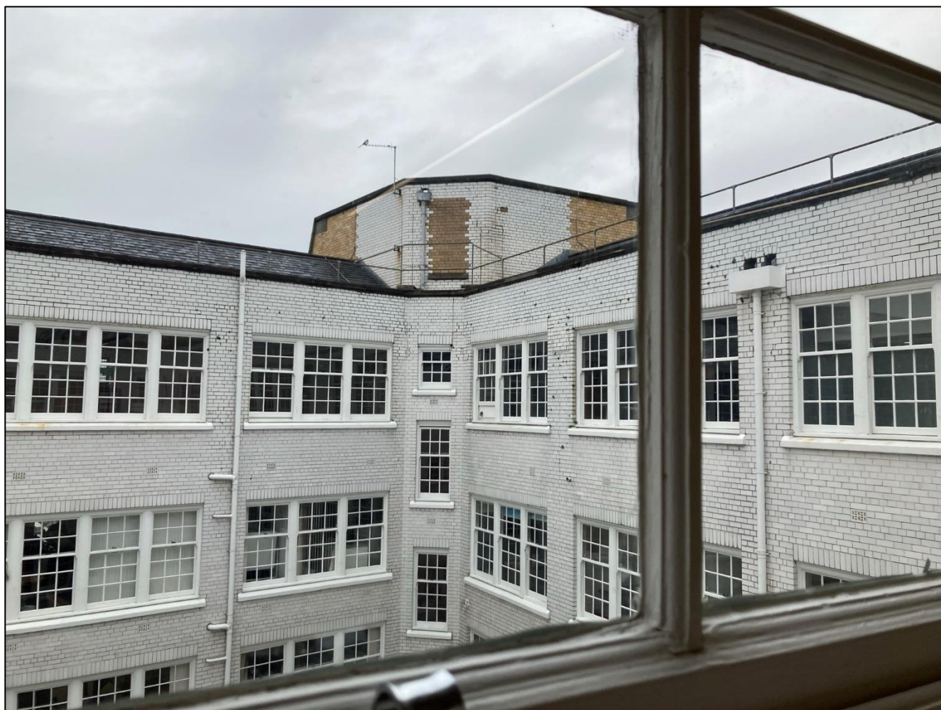
View into lightwell from the thirteenth floor
