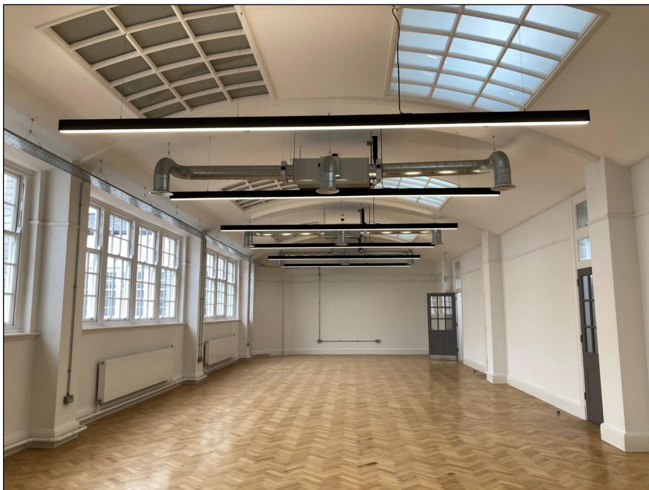
Thirteenth floor original parquet flooring and barrel ceiling; wall nibs and doors denote original partitions
