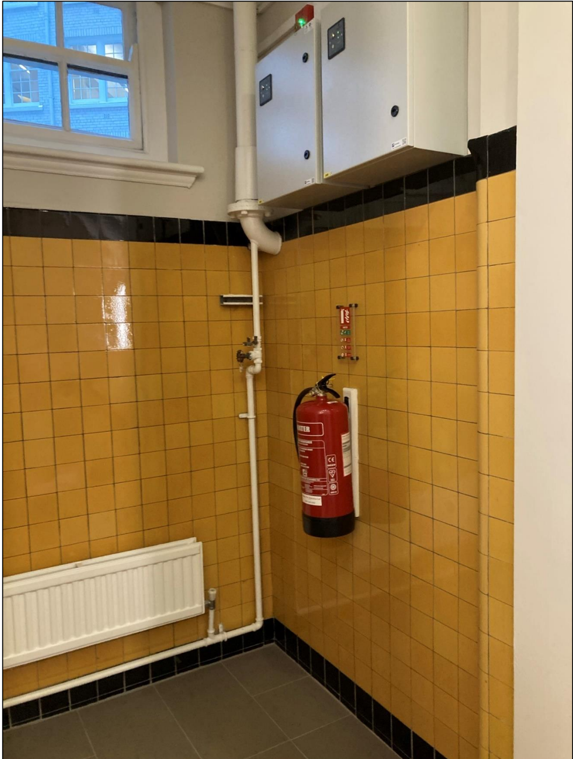
Original tiling in stairwell
