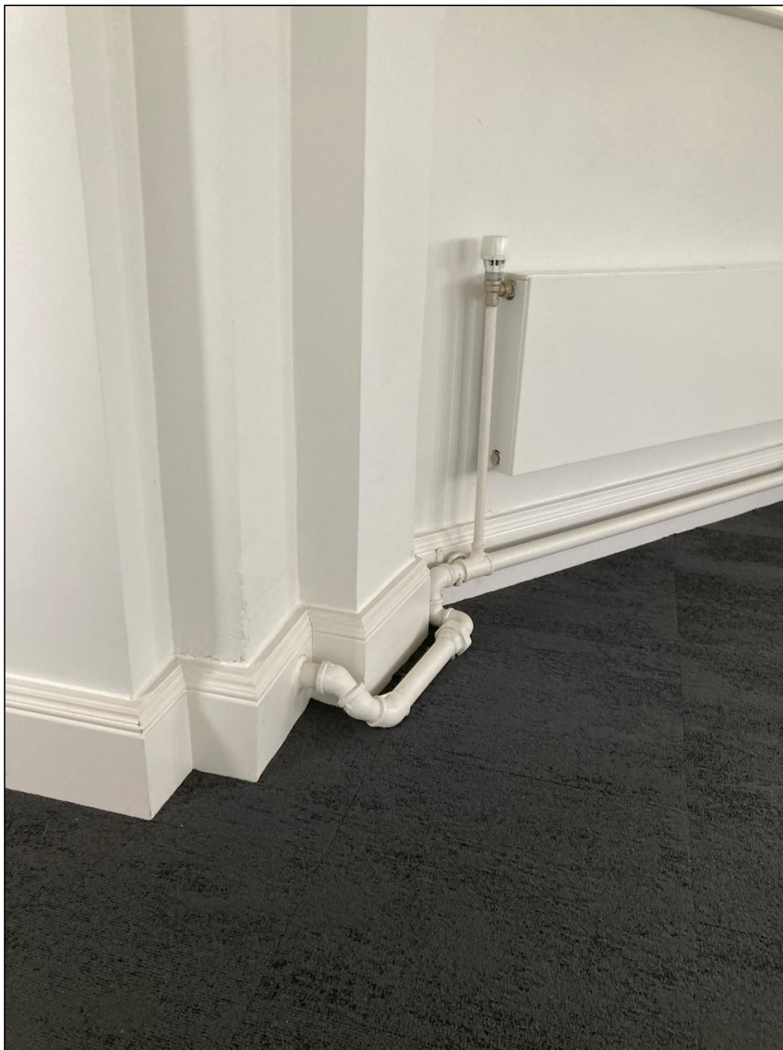
Thirteenth floor carpet and skirting (likely non-original)
