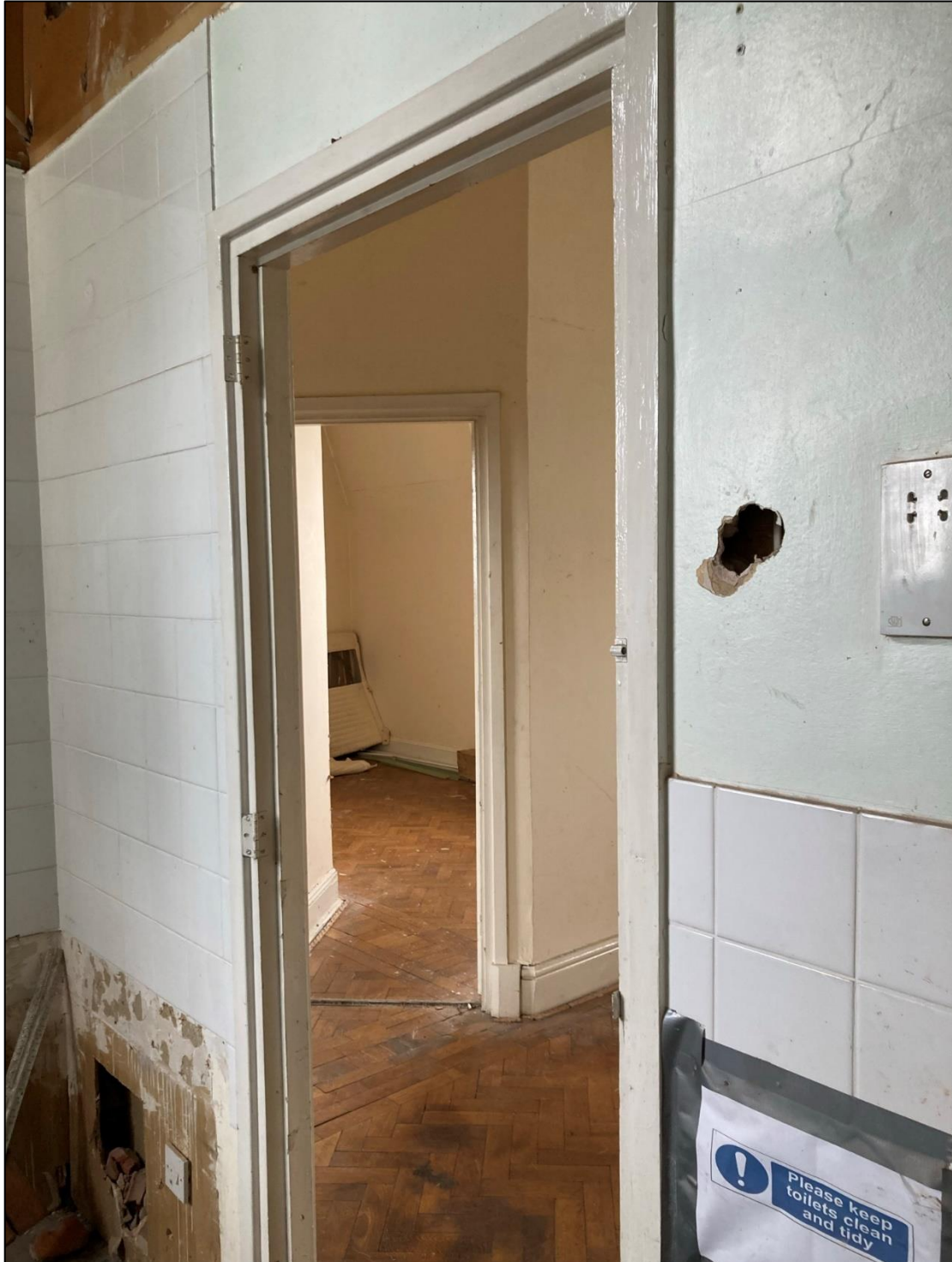
Original parquet flooring, caretaker's flat
