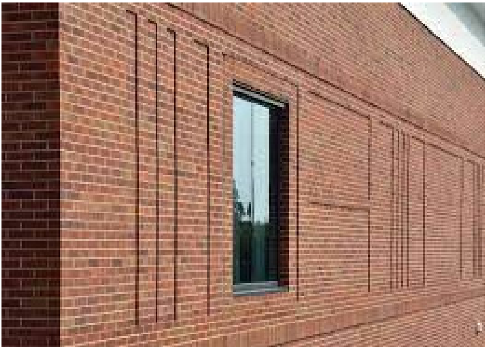
RECESSED BRICKWORK PANEL
