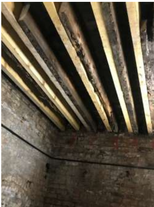
Photograph no.14 : Existing floor joists retained and spliced with new timber for support.
