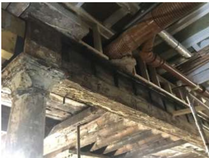
Photograph no.12: Existing beam and floor deck with new floor construction above.
