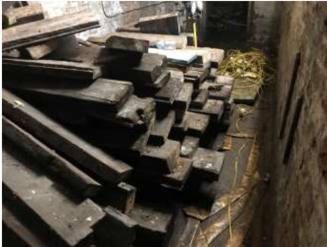
Photograph no.1: Stock Pile of existing rafters.
