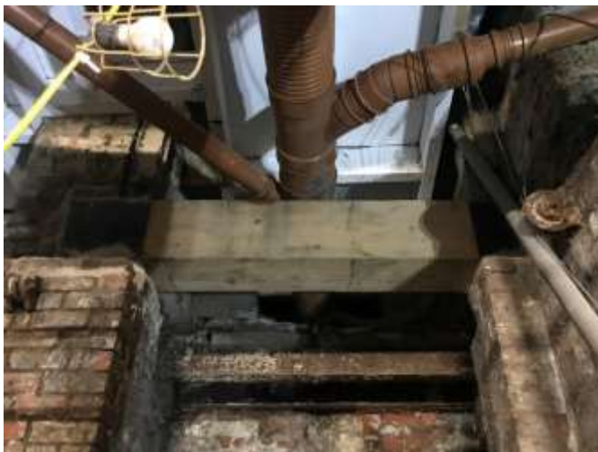
Photograph no.10: Complete beam Replacement with like for like `Douglas Fir`. Refer to Highlighted Section of drawing Ref: LK.01-102: Extents of Remedial Works to Existing Ground Floor Construction and also drawing ref: LK.01-101: Remedial Works to Existing Ground Floor Construction.
