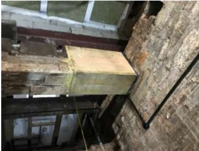
Photograph no.5: Splice Repair no.1.
