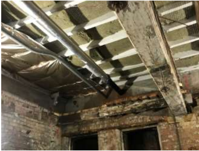
Photograph no.19: Showing Existing floor beam retained and the existing horizontal floor deck removed to allow access to the new floor structure.
