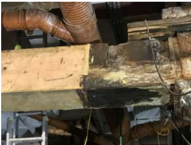
Photograph no.6: Splice Repair no.2.
