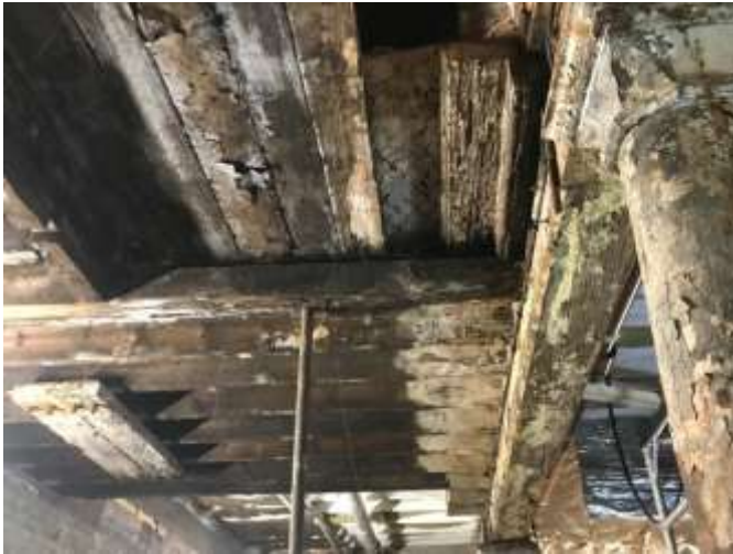
Photograph no.15: Existing floor beams and joists retained.
