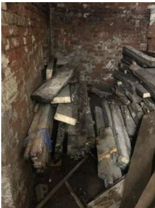
Photograph no.2: Stock Pile of existing rafters.
