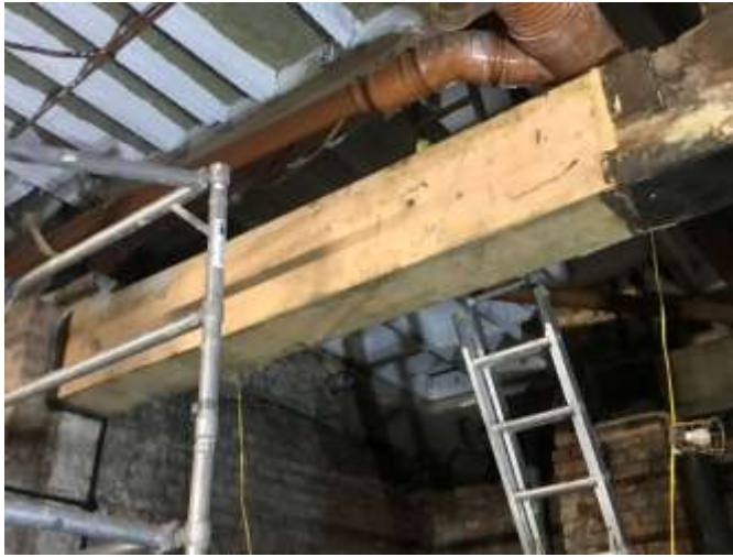
Photograph no.7 : Splice Repair no.2.
