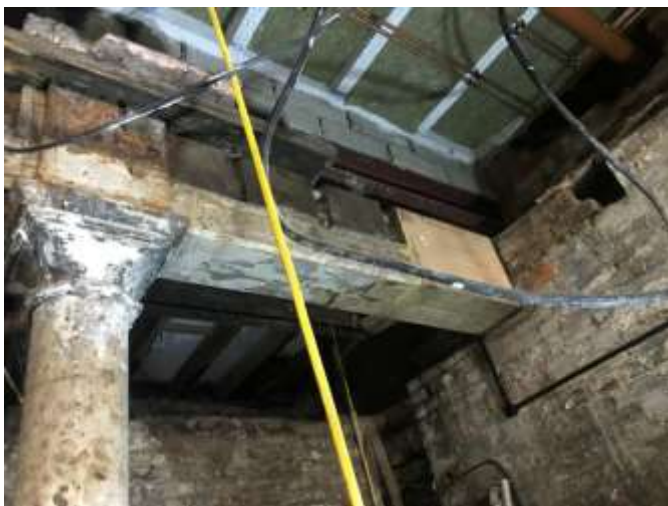
Photograph no.4: Splice Repair no.1.
