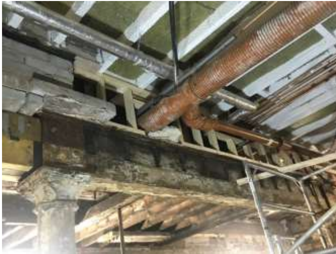
Photograph no.11: Existing beam and floor deck with new floor construction above.
