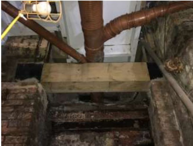
Photograph no.9: Complete beam Replacement with like for like `Douglas Fir` Refer to Highlighted Section of drawing Ref: LK.01-102: Extents of Remedial Works to Existing Ground Floor Construction and also drawing ref: LK.01-101: Remedial Works to Existing Ground Floor Construction.
