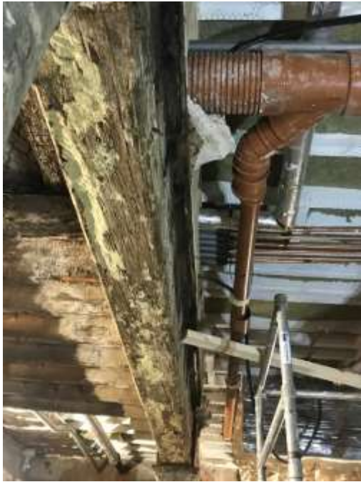
Photograph no.13: Existing beam ref A with putty treatment as installed by PRS.
