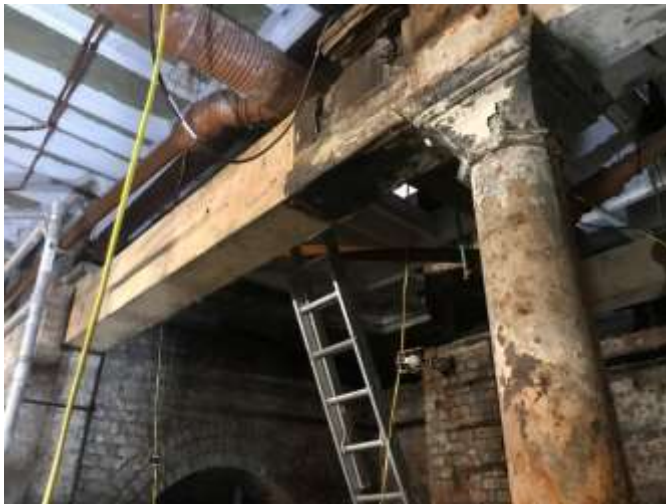
Photograph no.8 : Splice Repair no.2.
