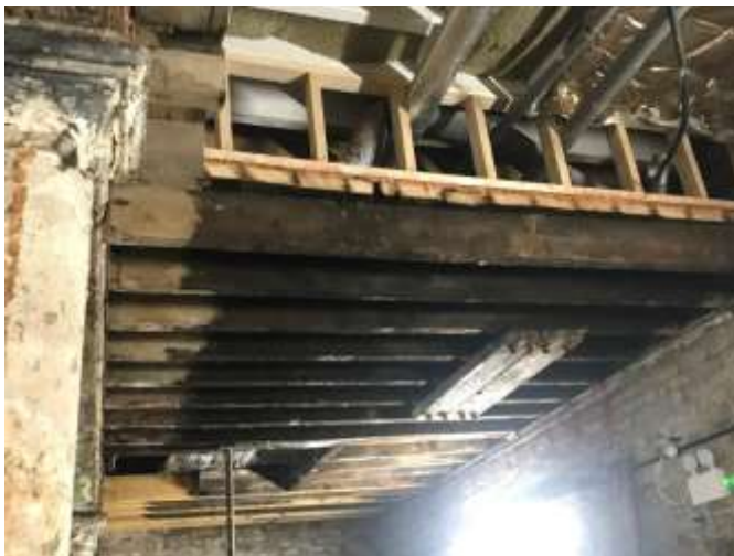
Photograph no.16: Existing floor beams and joists retained.
