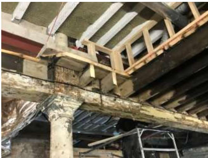
Photograph no.18: Showing Existing floor beams and joists that are to be retained and to be underdrawn with 2no. layers of 12.5mm plasterboard to provide basic fire protection.
