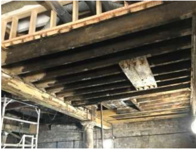
Photograph no.17: Existing floor beams and joists retained.
