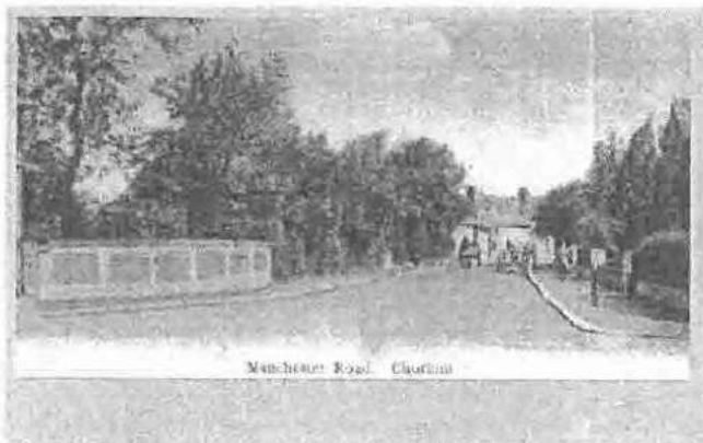
Plate 2. Manchester Road c.1900 (with barn in background!)
