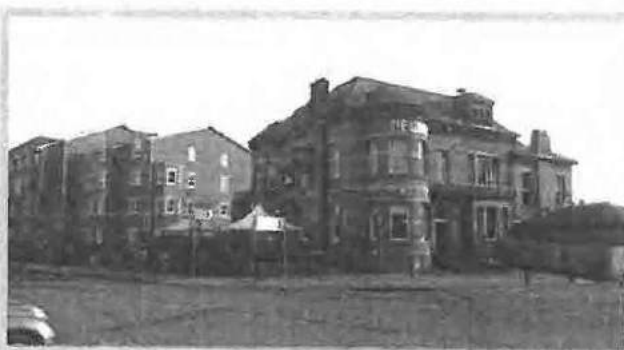
Plate 7. The listed Loyd's Hotel and recent large apartment block adjacent
