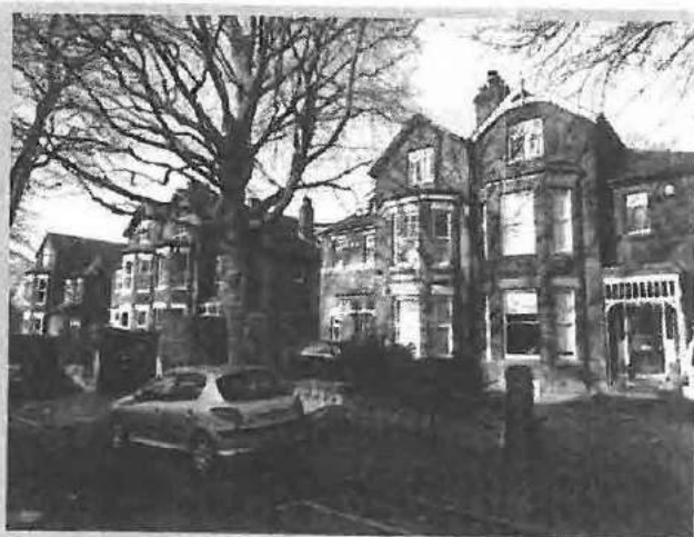
Plate 14. Opposite side of Vincent Avenue
