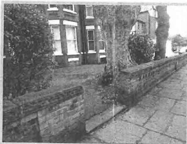
Plate 13. Brick-panelled front boundary wall with stone coping
