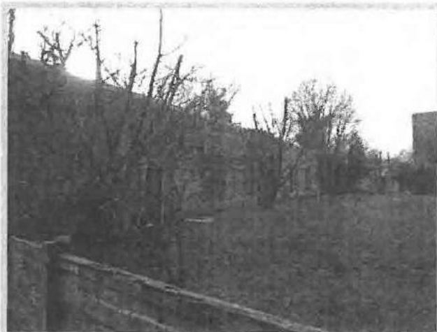
Plate 17. Rear boundary wall
