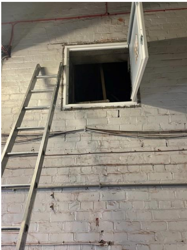
Photo 2. Existing access to roof void.
