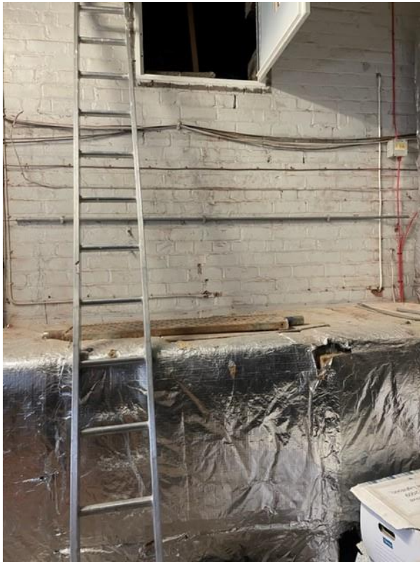
Photo 1. Existing access to roof void.
