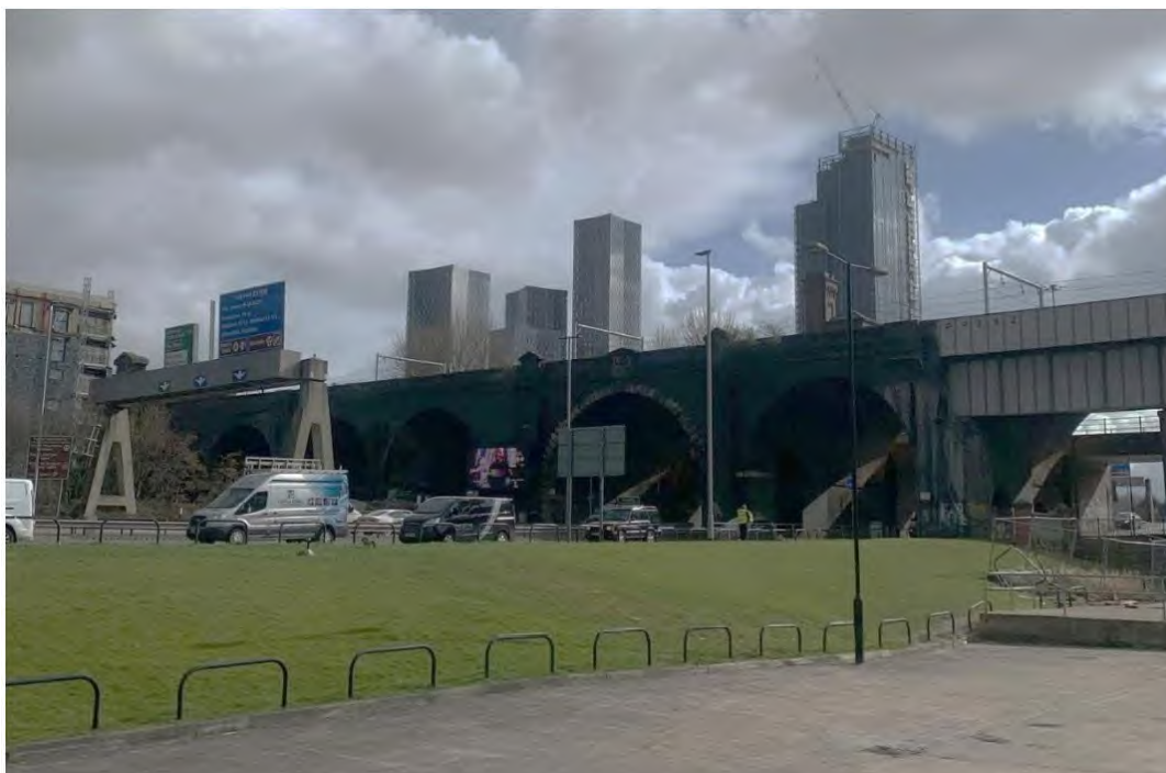
Figure 4.2: Castlefield Railway Viaduct From G-Mex to Dawson Street (Authors Own, 2021)
