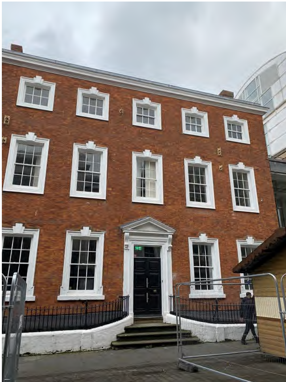
35 And 37 King Street and Attached Railings
