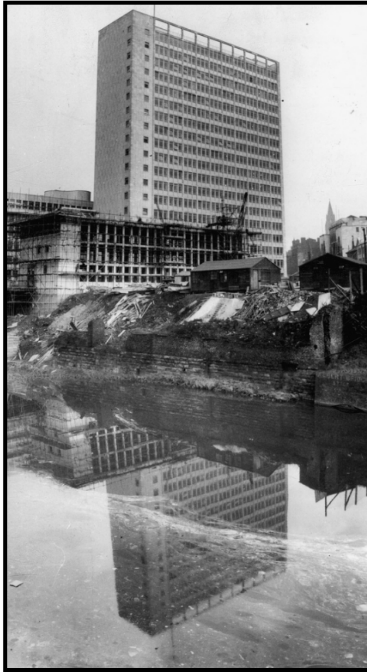
Figure 3.14: View east from Salford, with the low-rise section of Albert Bridge House under construction, c.1959. The pollution in the Irwell is extremely visible.
