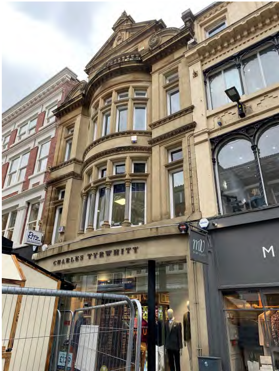
Warehouse Shop (Authors Own, 2022)
