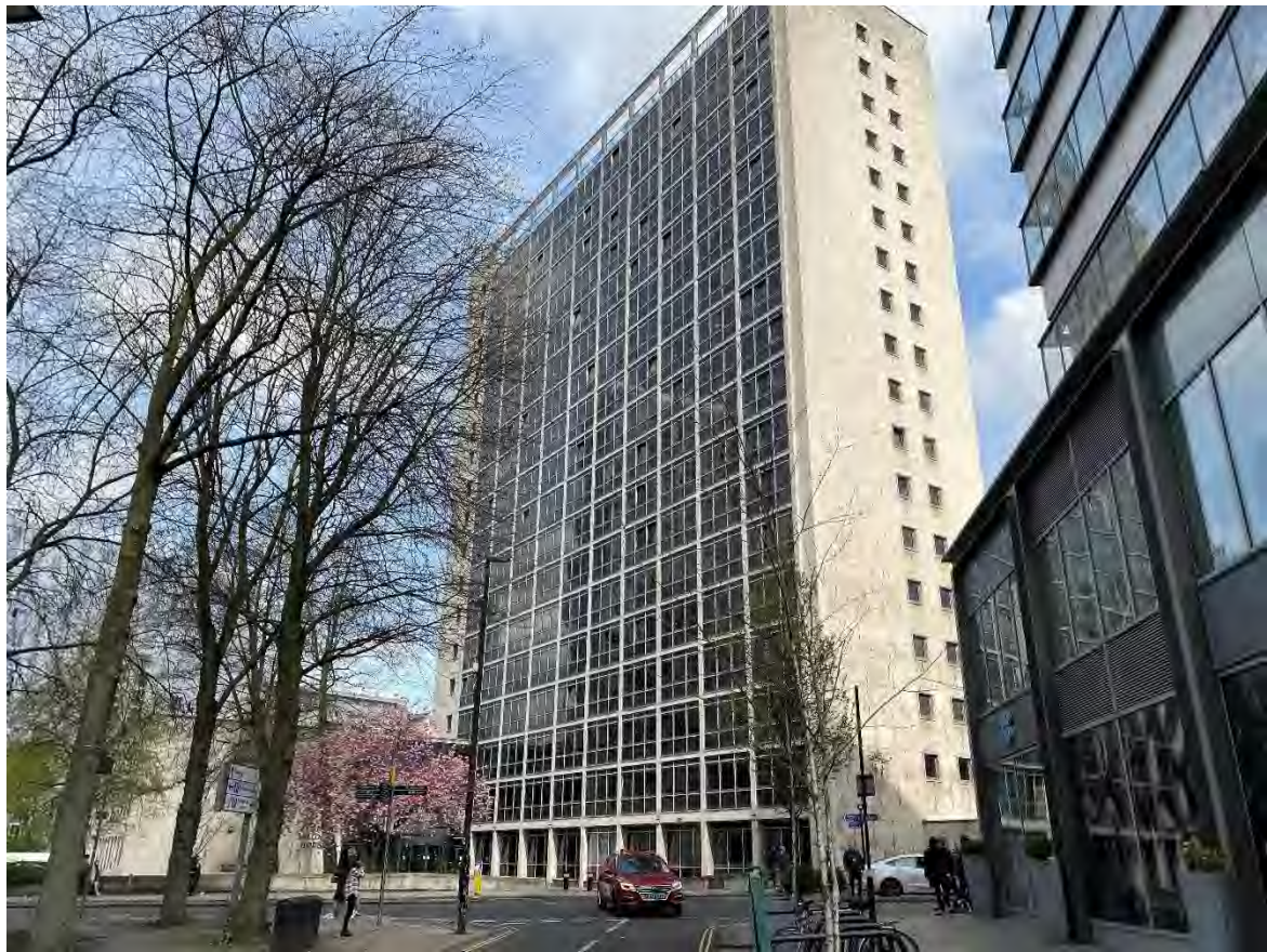
Albert Bridge House (Authors Own, 2022)
