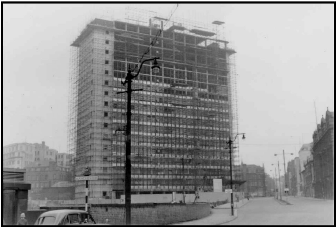
Figure 3.13: Construction of Albert Bridge House, showing the Masonic Hall to the right, c.1958
