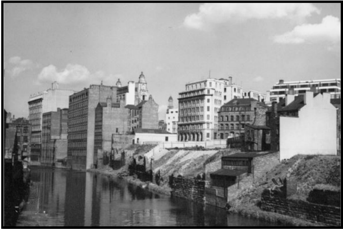
Figure 3.12: The Site on the right of the river prior to construction with hoarding erected, c. 1957. 3 St Mary's Parsonage is clearly visible.
