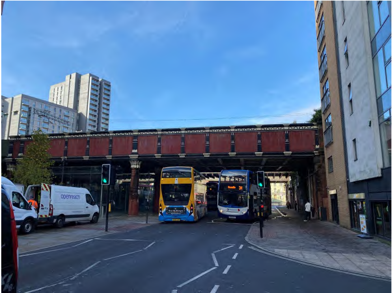
Southern Railway Viaduct and Colonnade (Authors Own, 2022)
