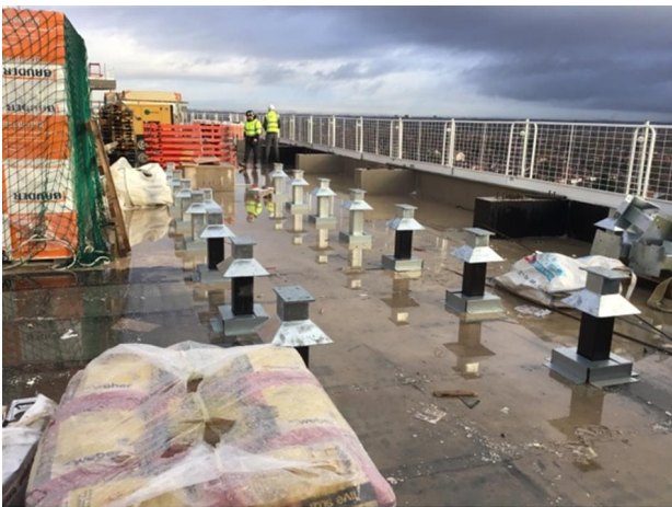
Photo 3 - View of level 9
