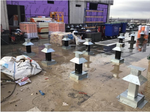
Photo 1 - View of progress to level 9
