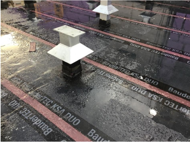
Photo 7 - View of steel supports
