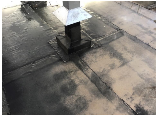
Photo 6 - View of AVCL to steel supports
