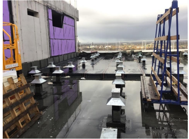
Photo 2 - View of progress to level 9
