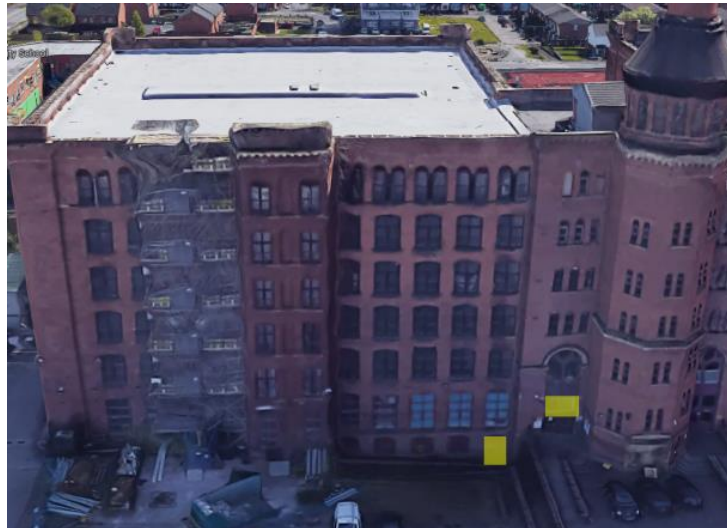
Figure 28. Ground & basement access
