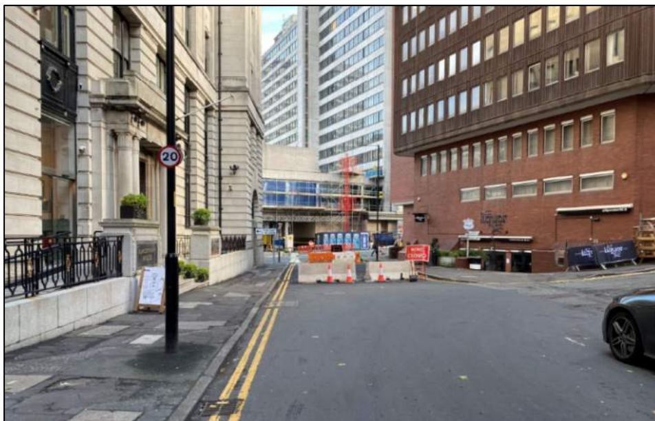
Figure 2.3 – Closure of St Mary's Parsonage at its Junction with Blackfriars Street
