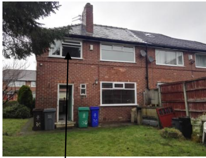
Rear of no. 30 Melling
