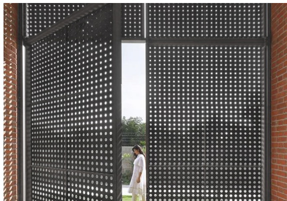
7. BLACK STEEL PERFORATED GATES & SIGNAGE
