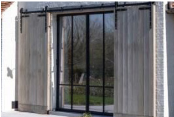
2. TIMBER SLIDING SHUTTERS
