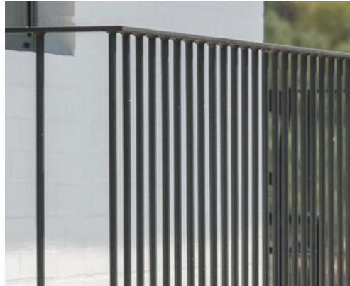
3. POWDER COATED STEEL BALUSTRADE
