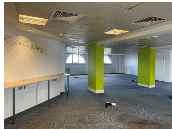
Figure 17: View towards the front of the building (facing King Street). Original columns, beams and later arched windows visible, but all finishes are modern
