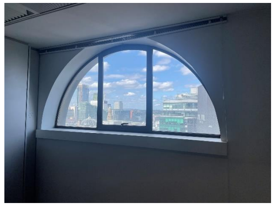
Figure 18: One of the arched 'Diocletian' windows which are located on the front elevation. Not part of the original design and not evident on early photographs
