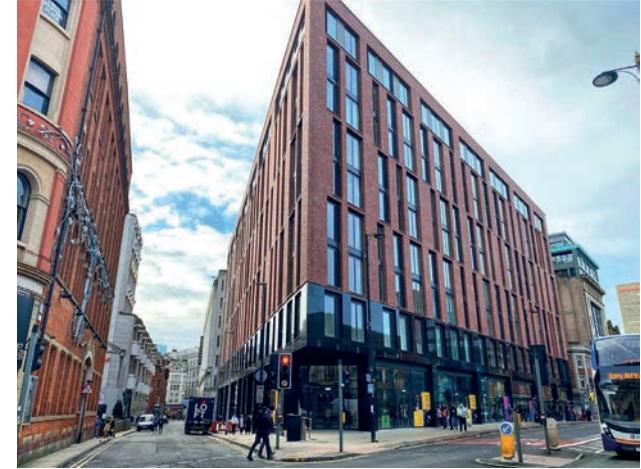
3. Transmission House (Completed 2020)
