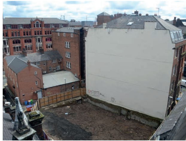
12. Overall view of the vacant site.
