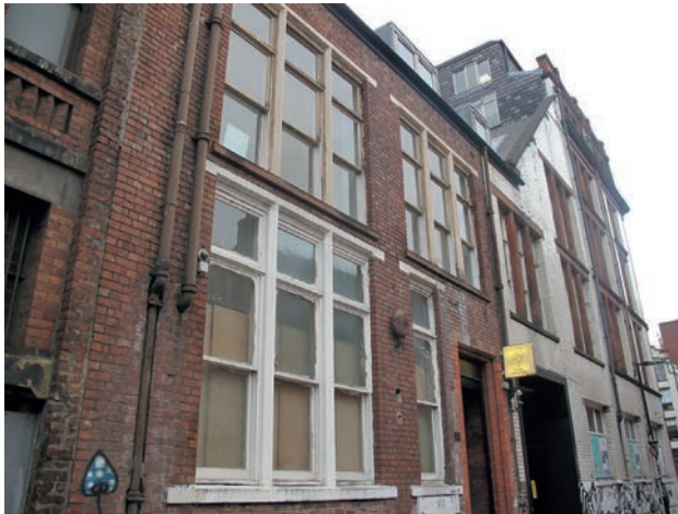
7. View of 22 Dale St. (Grade II Listed) from Little Lever Street.
