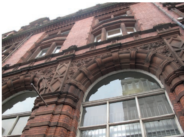
11. Details of 22 Dale Street (Grade II Listed)
