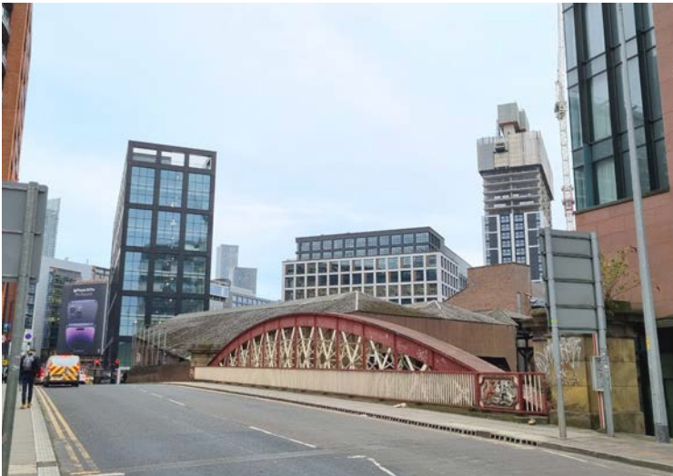
2. VIEW FROM IRWELL ST.
