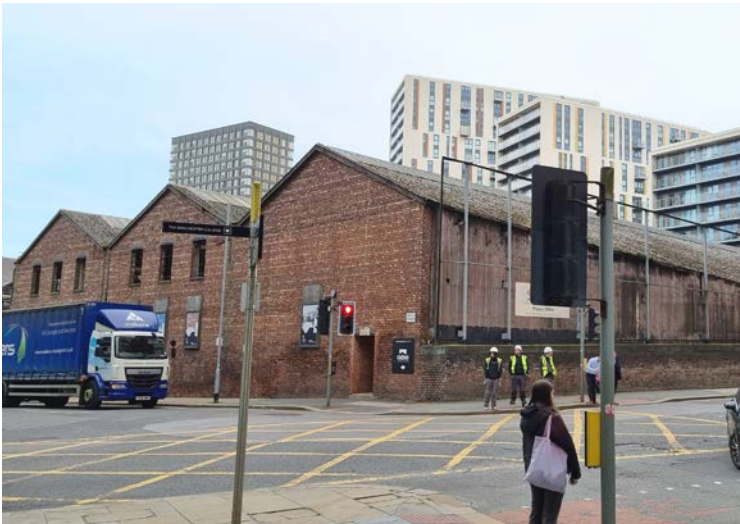
1. VIEW FROM CORNER OF WATER ST. AND NEW QUAY ST.
