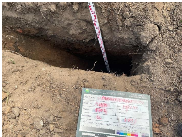
Trial Pit 2: Internal view of excavation
