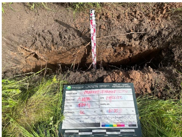
Trial Pit 1: Internal view of excavation
