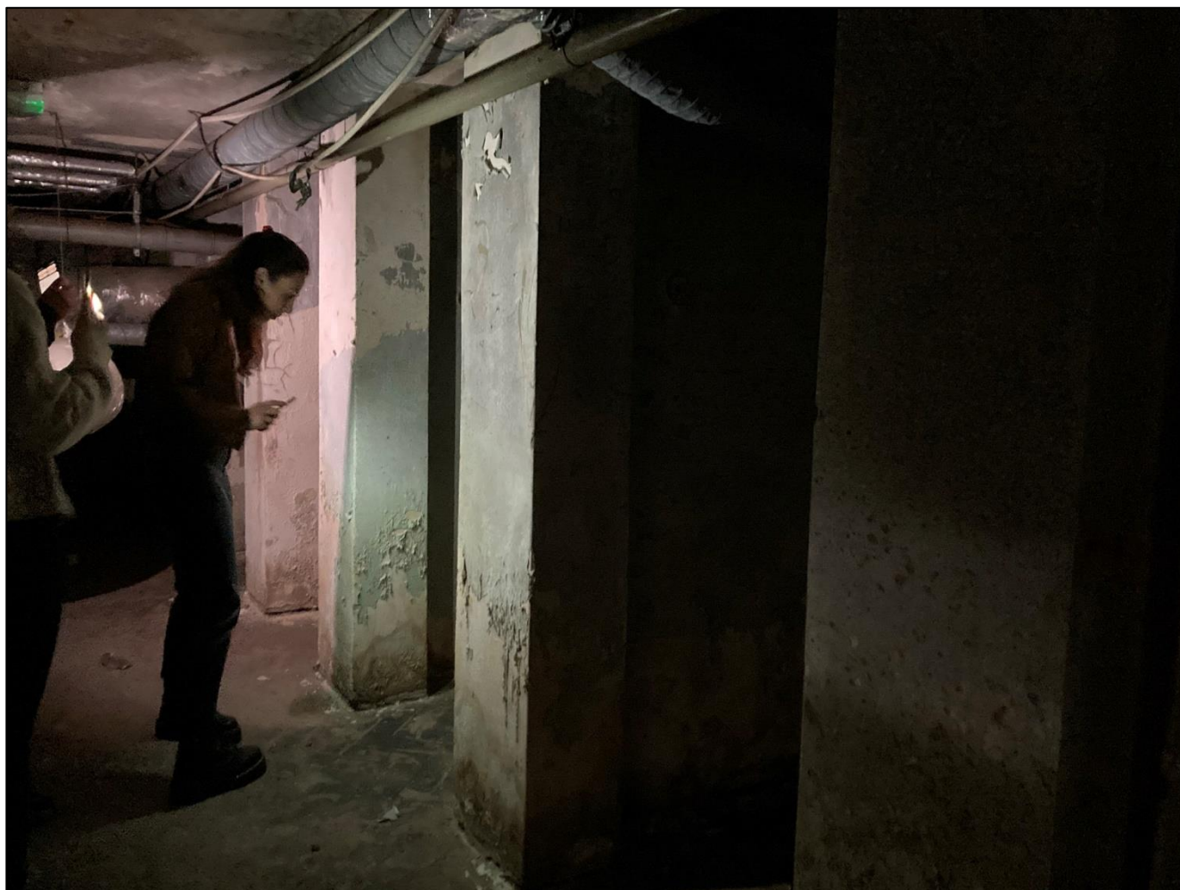
Existing service space below the pool, with partitions originally used for changing/treatments
