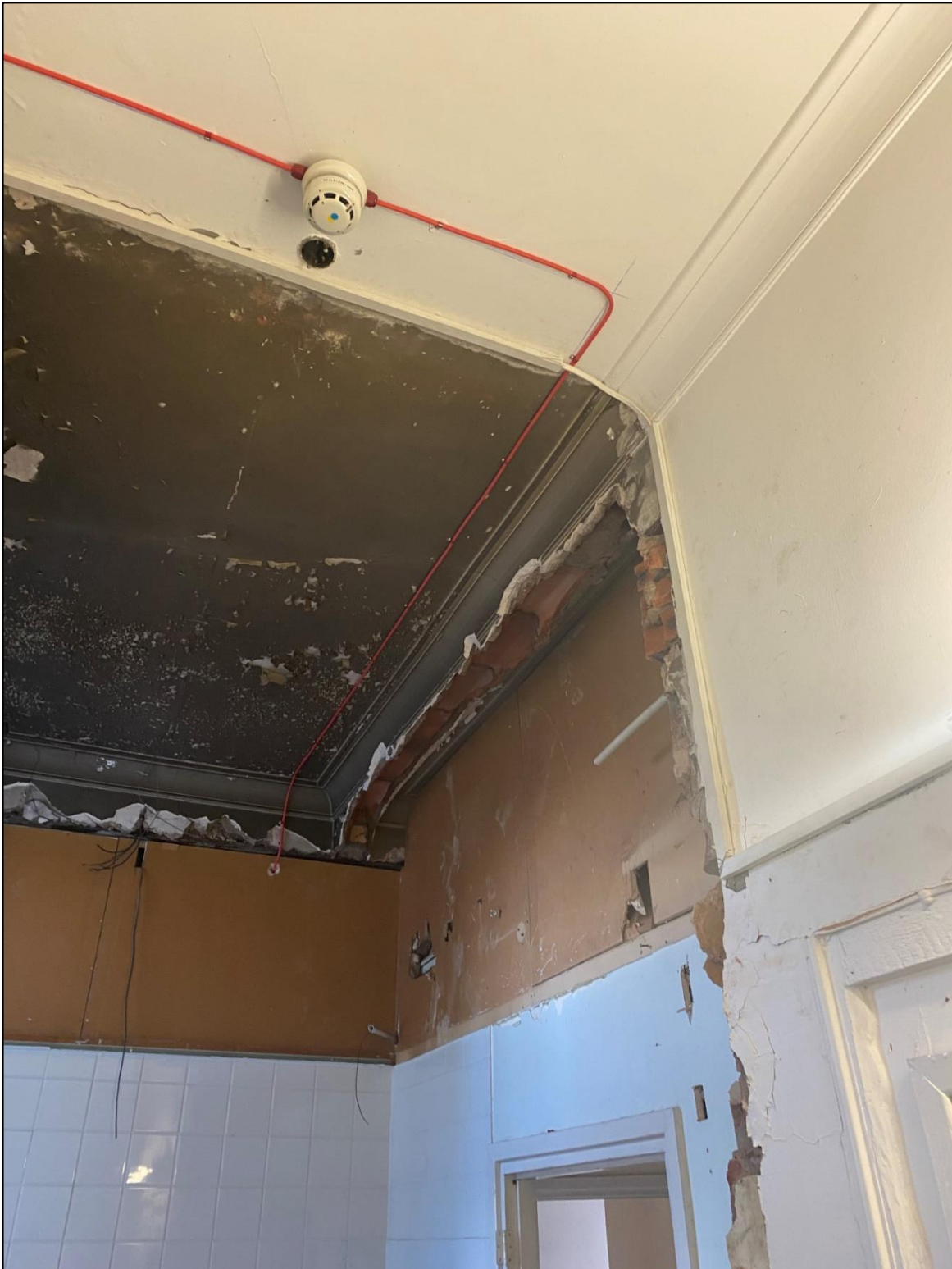
Caretaker's flat showing original position of wall
