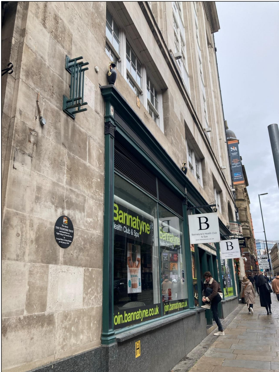
Quay Street façade
