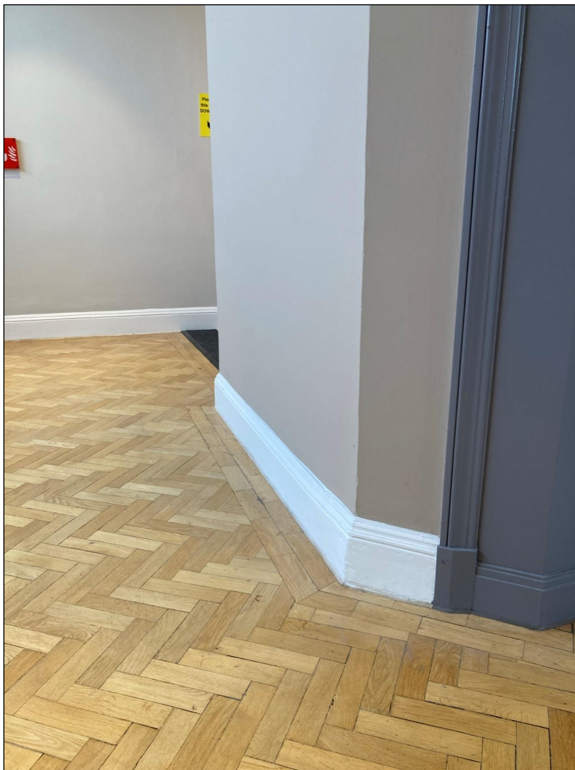
Original parquet flooring and skirting, thirteenth floor
