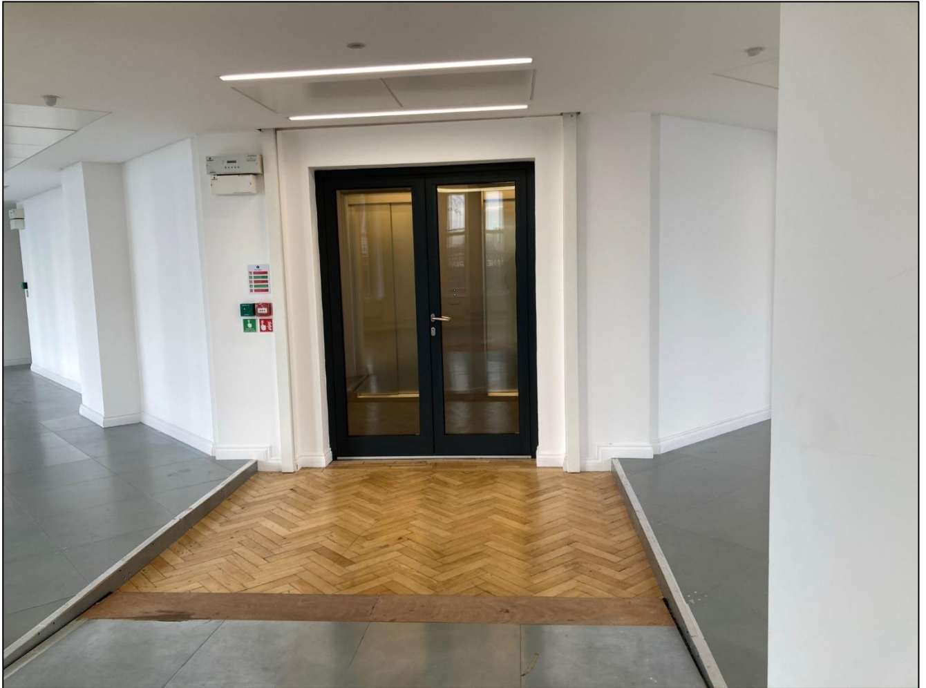
Original parquet flooring to entrance door, eighth floor
