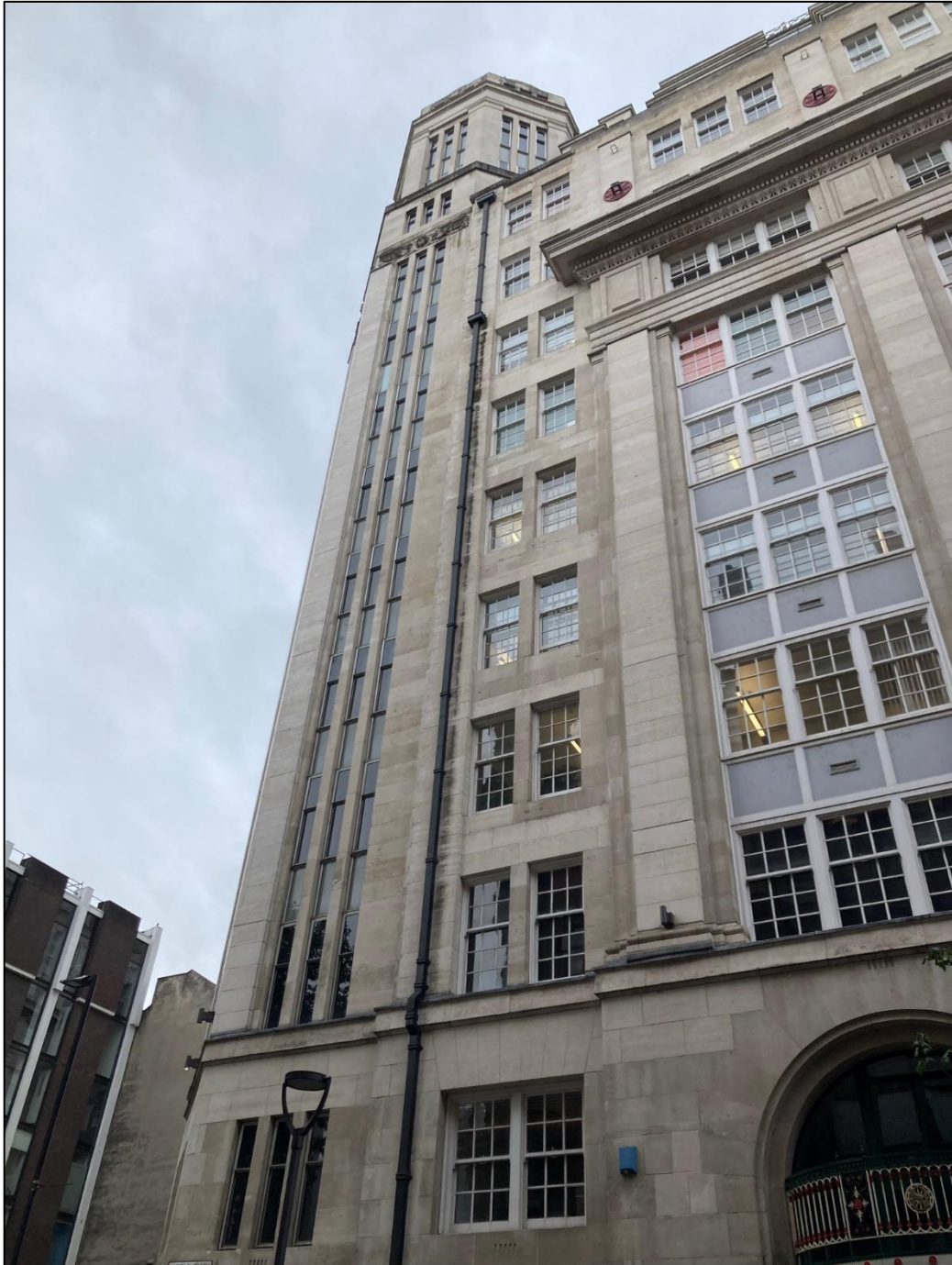
Corner tower to Quay Street
