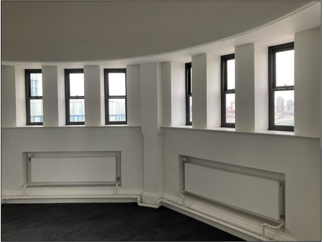
Corner tower to thirteenth floor
