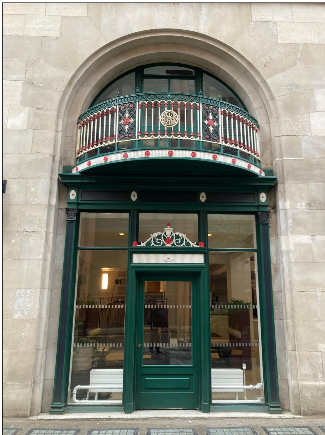
Original decoration to Little Quay Street façade
