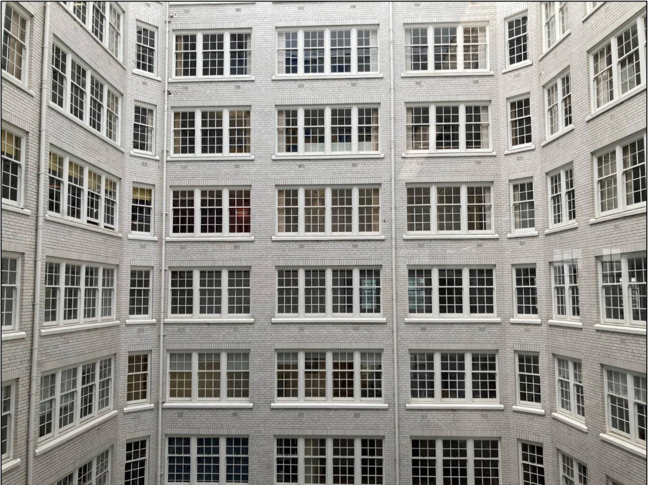
View of lightwell from eighth floor
