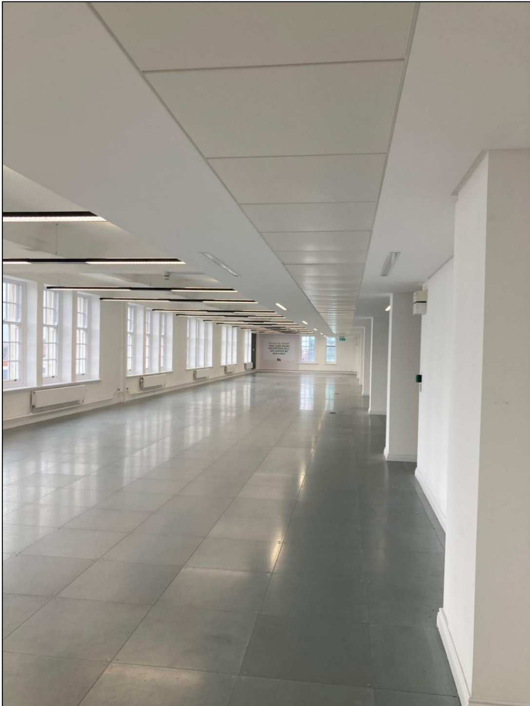
Non-original dropped ceiling (right), exposed original coffered ceiling (left), eighth floor
