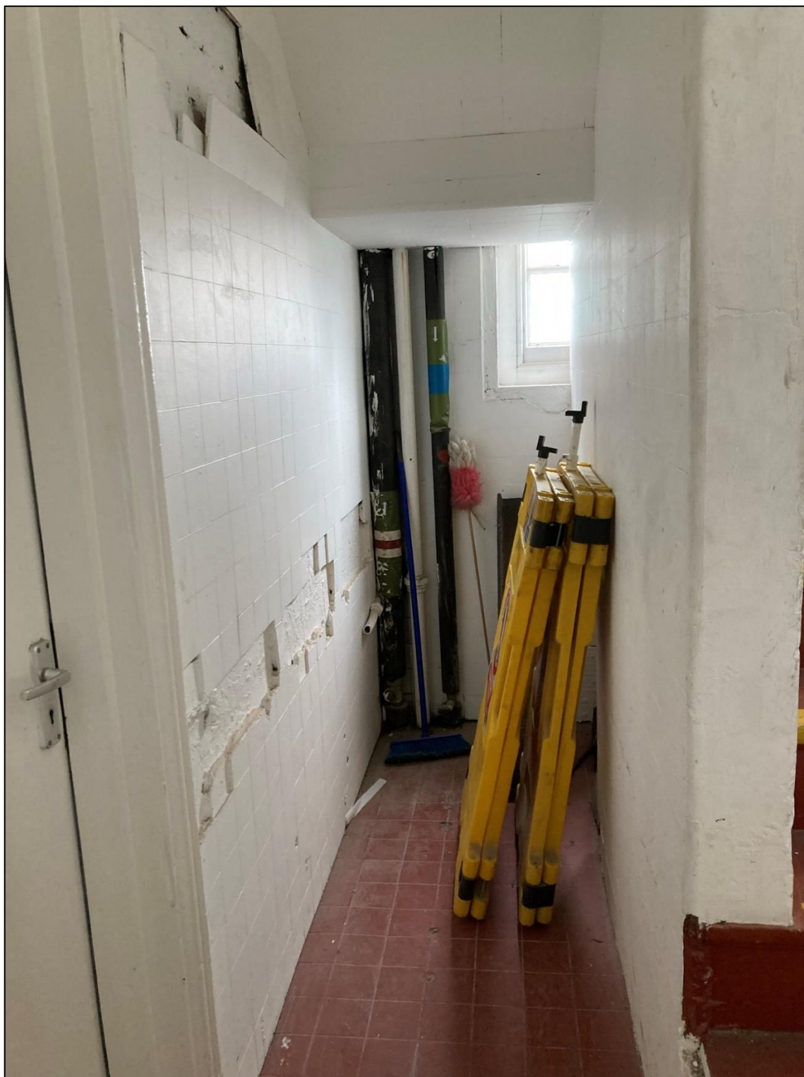
Entrance to caretaker's flat
