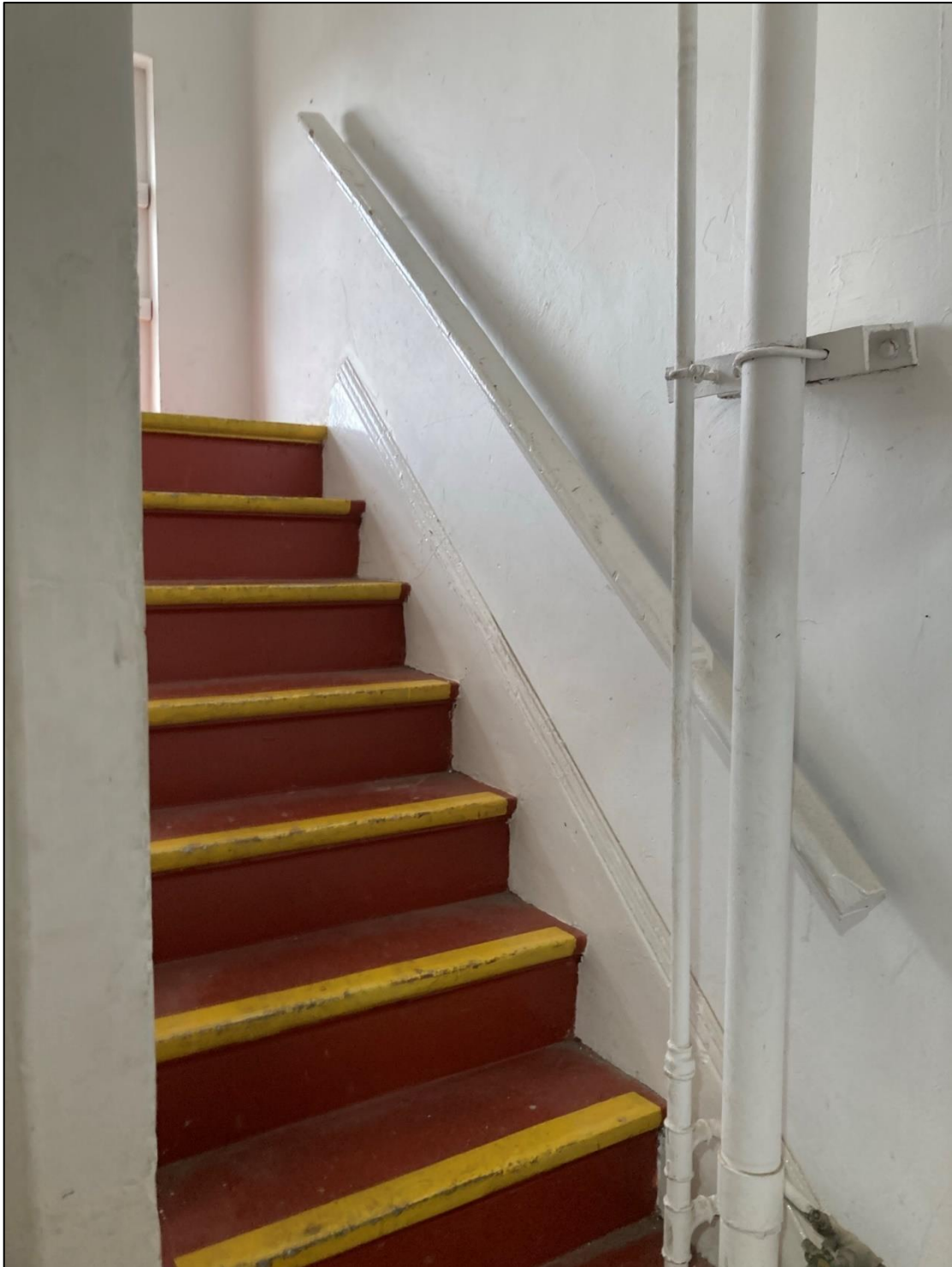
Stairs up to caretaker's flat
