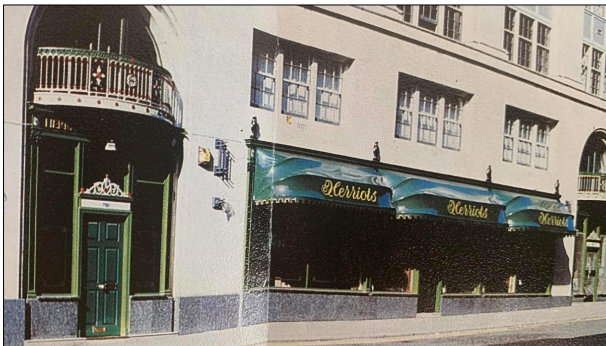
Figure 16 – 1980's image of Quay Street elevation, showing canopies above the window openings with Herriots lettering, as well as the paint scheme to the metalwork which exists today.
