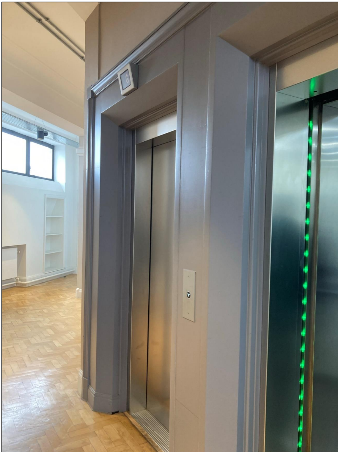
Original parquet flooring and lift surrounds, thirteenth floor
