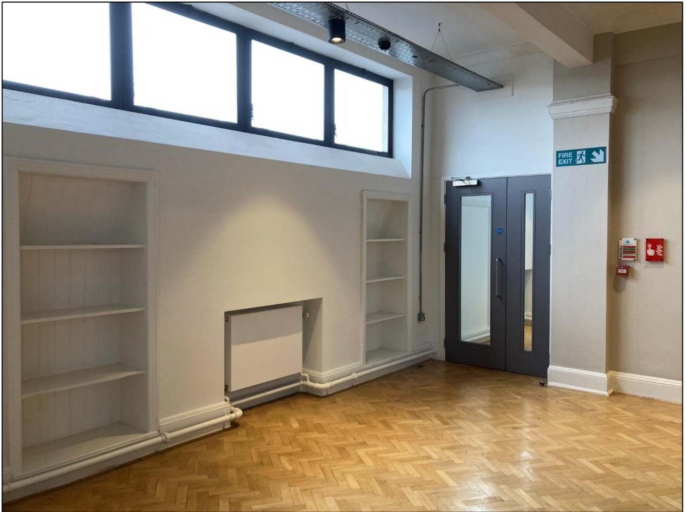
Original parquet flooring, thirteenth floor
