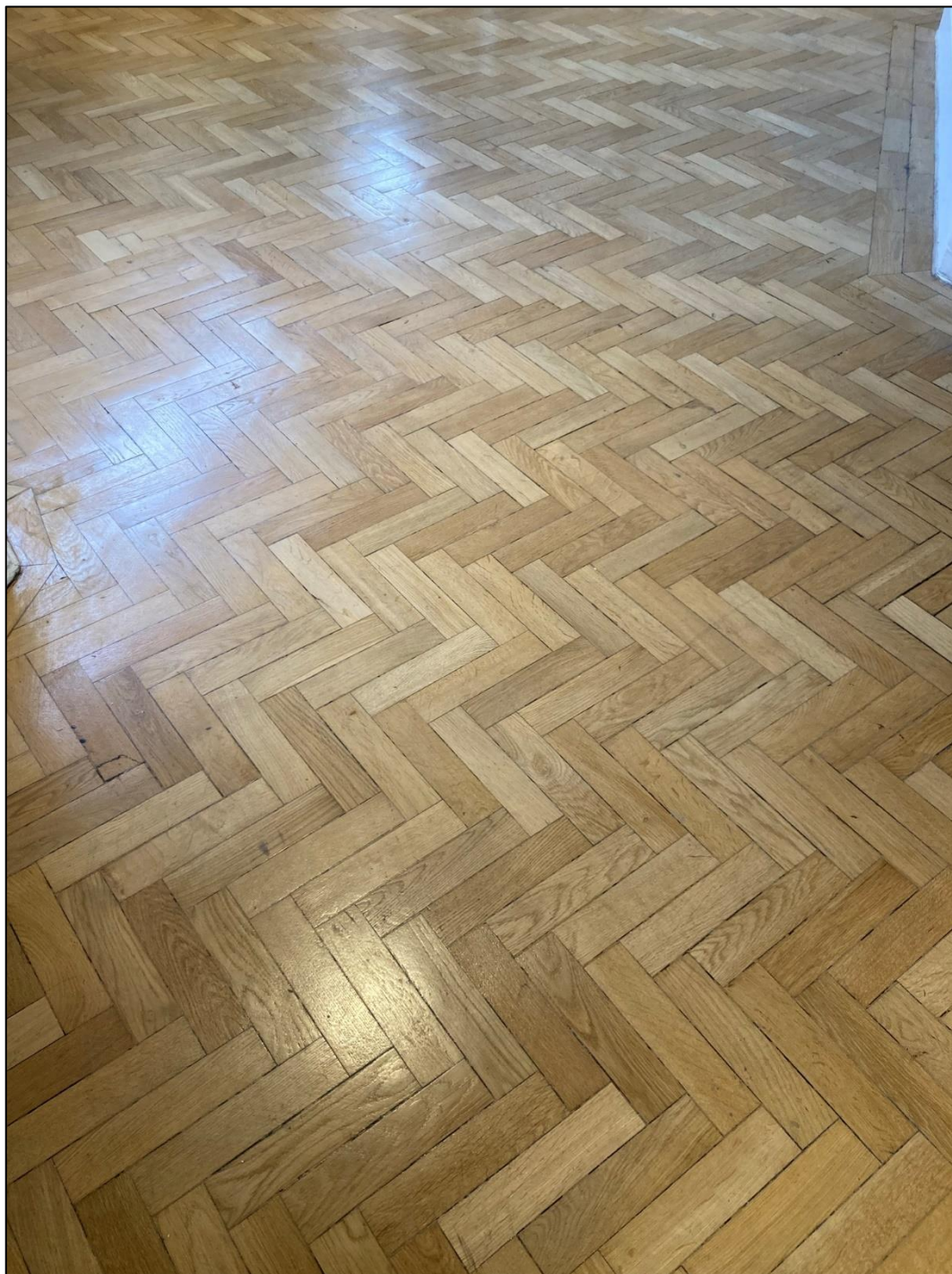
Original parquet flooring, thirteenth floor
