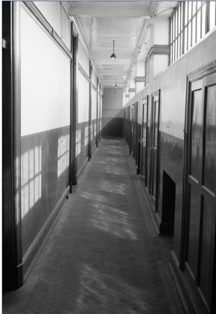
Figure 33 – Thirteenth floor corridor (1958)
