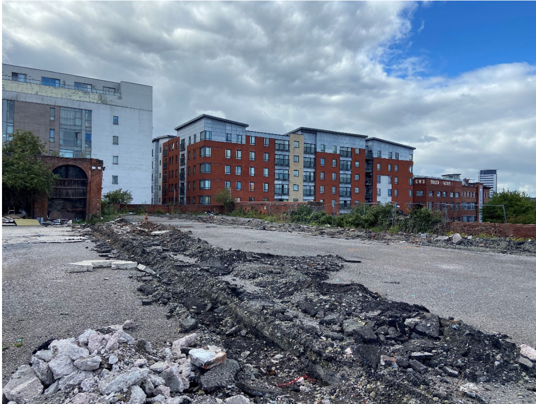
Photograph 3 – North west area of site, showing previous geophysics survey
