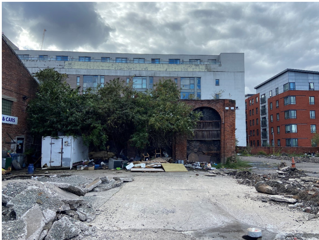
Photograph 4 - West of site showing adjoining boundary wall
