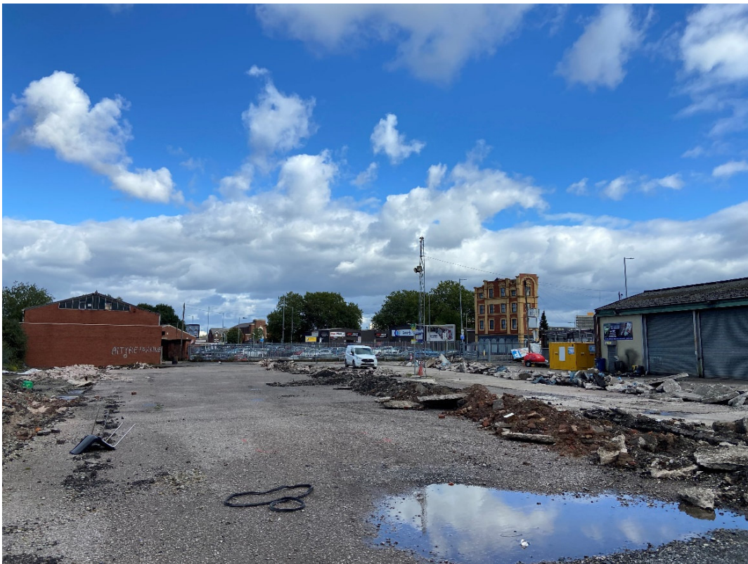
Photograph 6 – Overview of site area
