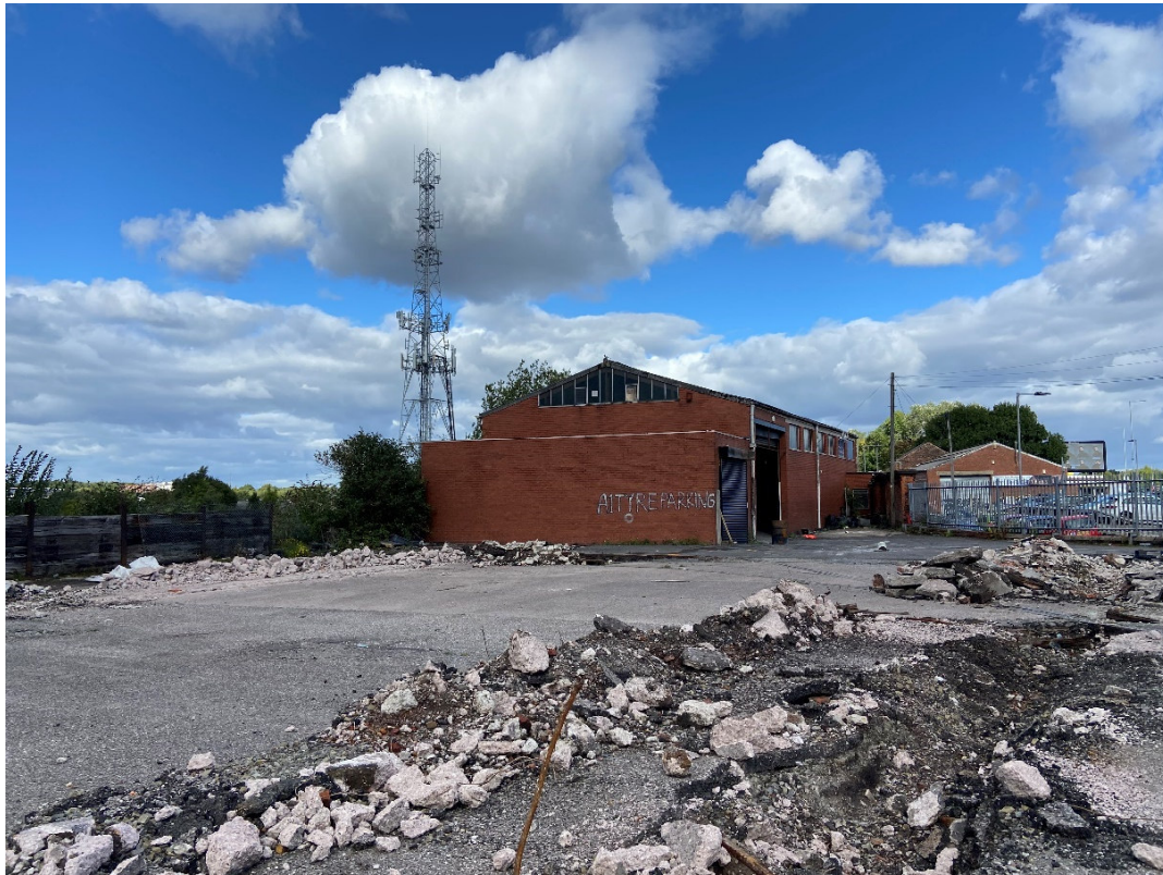
Photograph 1 – East of site showing existing warehouse building
