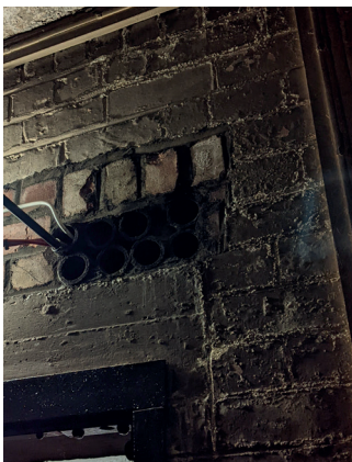
Existing cable routes into the basement to be reused.
