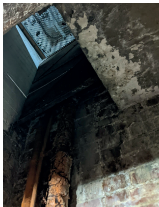
Existing cable routes into the basement to be reused.
