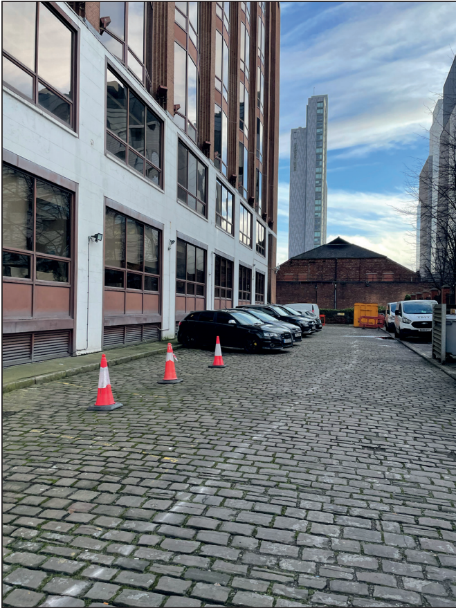
Photo of rear parking area and location of proposed EV charging points
