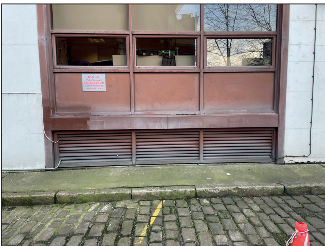
Photo existing louvres on the rear/east facade
