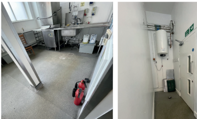
Photographs of the existing conditions with the function kitchen
