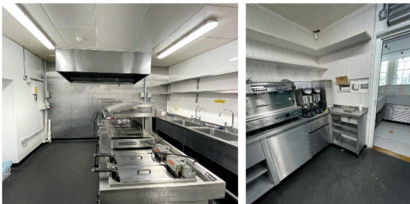
Photographs of the existing conditions within the cafe kitchen
