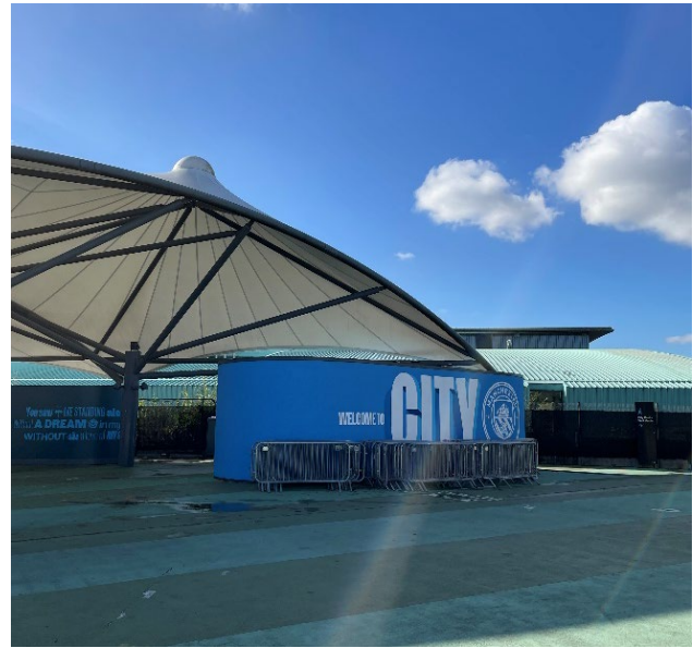
Figure 12 – Canopy 1 and associated structures
