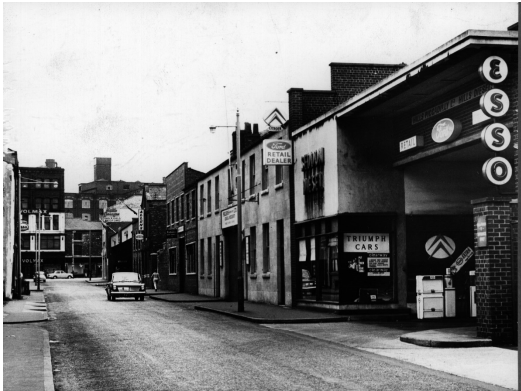
Figure 2.10: 1966 Photograph looking north-east along Port Street ©Manchester Libraries, Information and Archives. The full historic extent of 68 Port Street is shown, comprising a two-storey, seven bay width building with central entrance archway.
