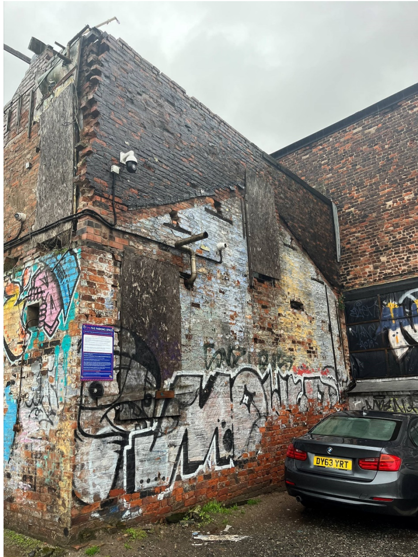
Figure 2.13: Rear, south-east elevation of 68 Port Street. The roof line of the former rear warehouse element of the building can be viewed within the brickwork. The rear of the building appears to have been subject to later alteration (with different brick type to the lower storeys). Slots for the roof joists of the arched cart entrance and building above can be seen in the north-west elevation of the building (left of image)
