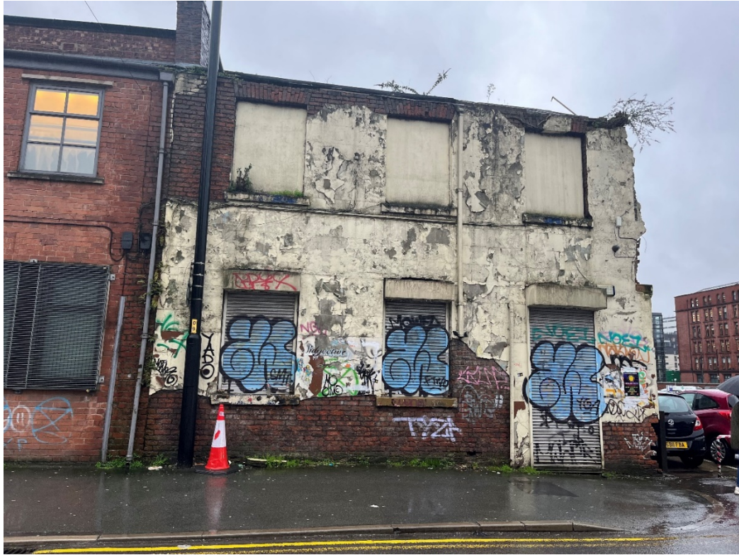
Figure 2.12: 68 Port Street as seen today from Port Street, looking south-east. The building adjoins one to the immediate north-east, known today as Sam's Yard. 68 Port Street has been altered at ground floor level by the insertion of rolling shutters and the removal of some of the render.
