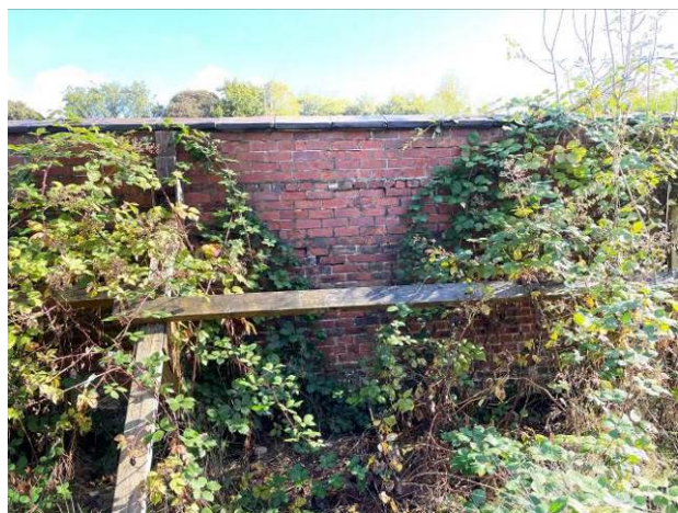
Differing bonding patterns to south (L) and west (R) walls. Note engineering bricks in upper area of west wall.
