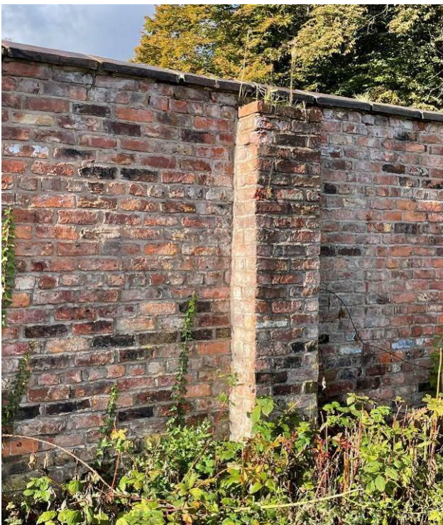
Brick piers to west (L) and south (R) walls. Difference in coursing (see left image) suggests later additions.
