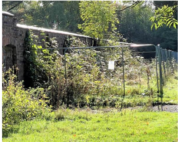
Area of the west boundary wall fenced off and supported by raking timber shores.
