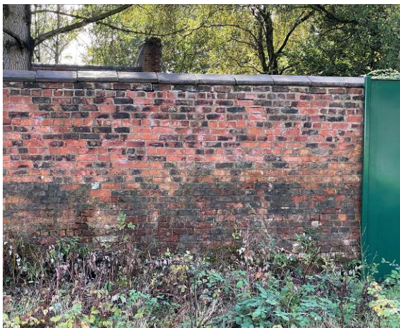
Differing bonding patterns to south (L) and west (R) walls. Note engineering bricks in upper area of west wall.
