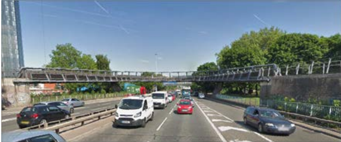
Figure 5.1: Footbridge over the A57 Mancunian Way
