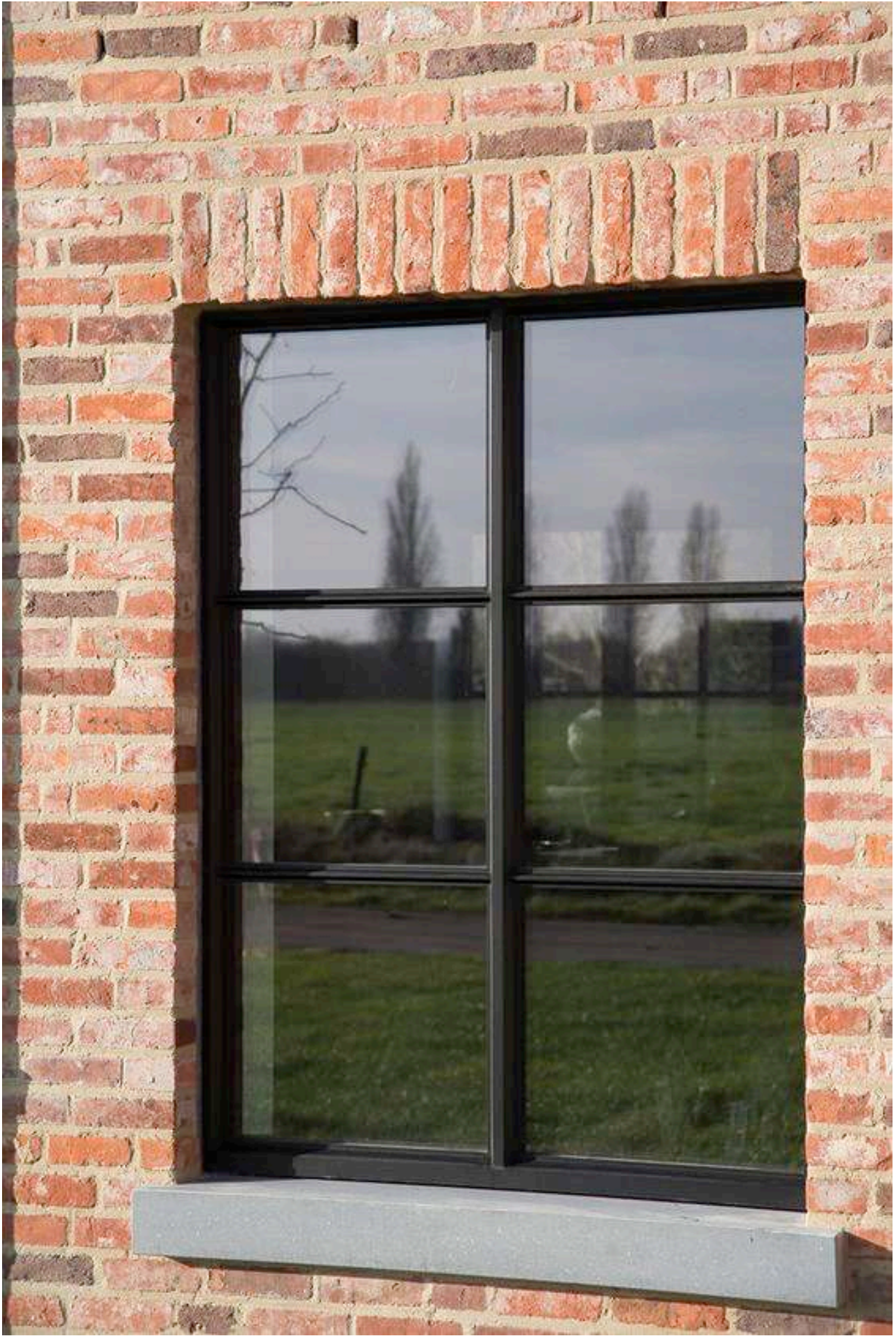
4. SLIMLINE PRECAST CONCRETE CILLS & COPING
