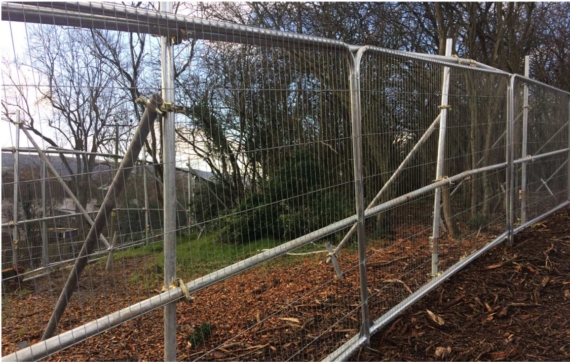
Above: Full specification barrier fencing.
