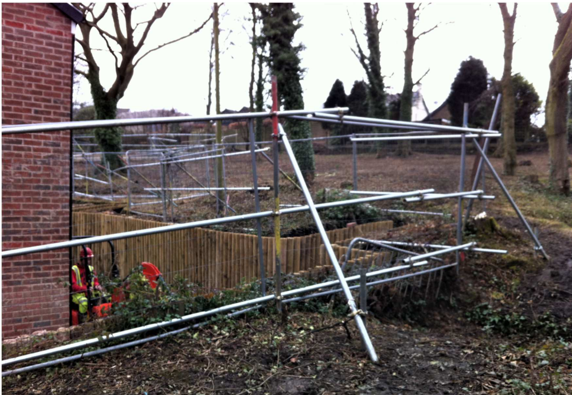
Below: Barrier fencing accurately placed adjacent variable and complex working zones.
