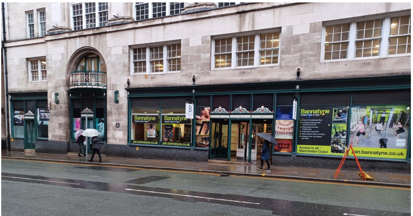
Photograph 1 Site as viewed from Quay Street source: case officer photograph taken 10.01.2022
