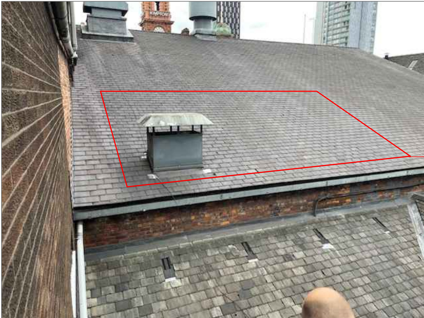
ROOF PENETRATION AREA FOR VENTILATION DUCT TO ENTER.
