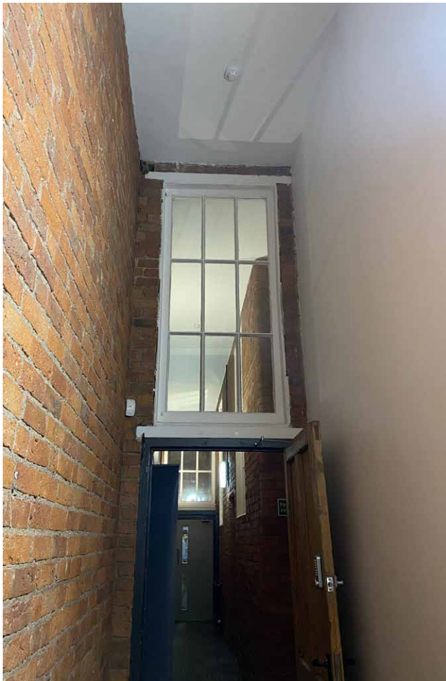
Some visible features from original design.
