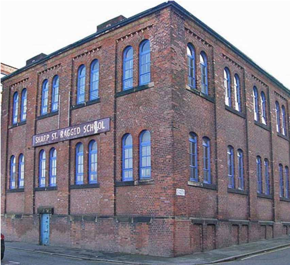
Sharp St Ragged School from the North showing the original building pre 2010 (before previous planning application and conversion to office)
