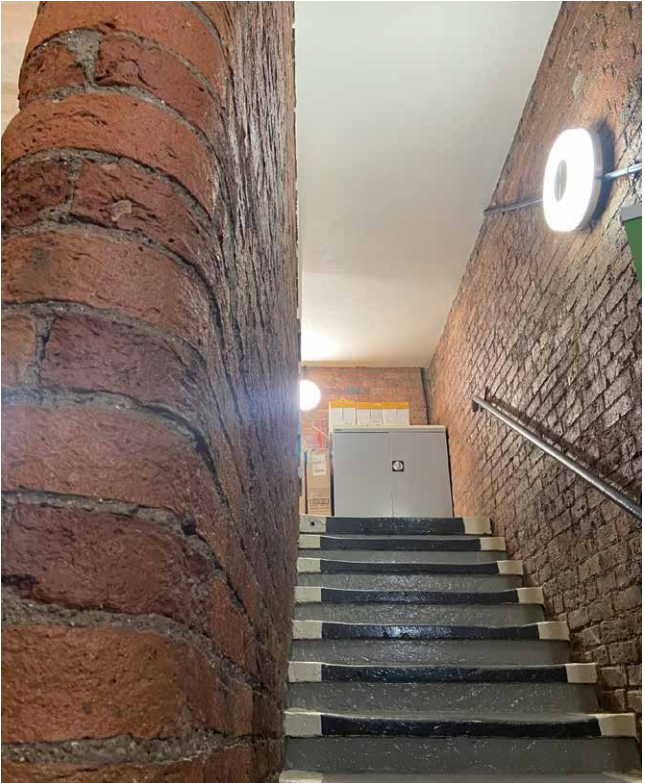
Secondary staircase, currently blocked off
