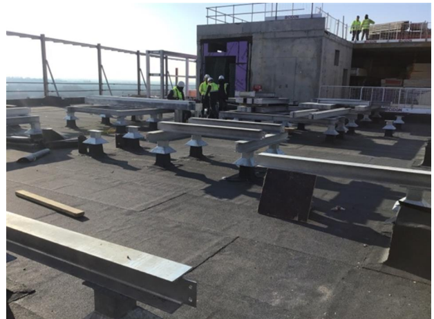
Photo 6 - Overview of section 3
