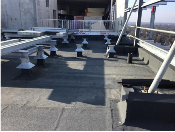
Photo 7 - View of cap sheet to section 3
