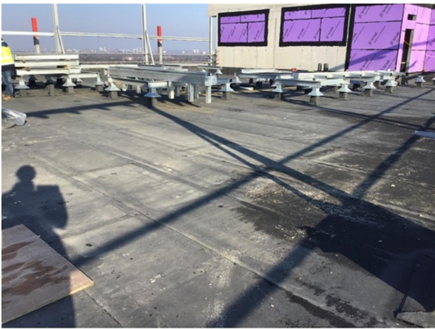
Photo 3 - Overview of level 9 section 3
