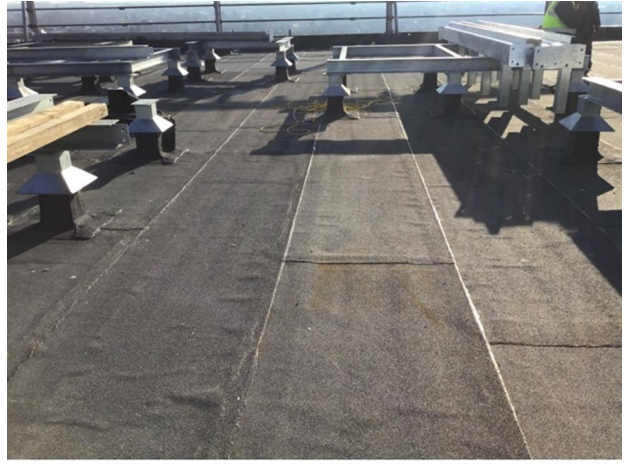
Photo 8 - View of cap sheet to section 3
