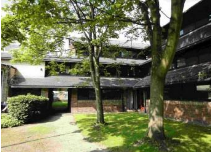
Photos of Ewings Building when viewed from the western side
