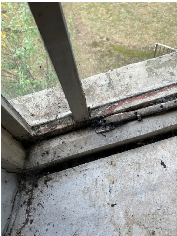
Existing window board
