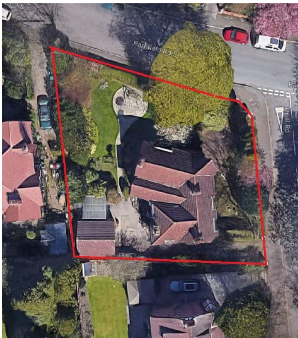
Figure 2. Aerial photograph of No.12 Parkfield Road South, with plot boundaries edged in red.
