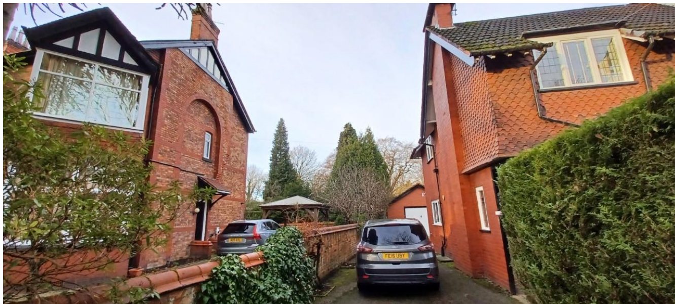
Figure 3. Photograph of the shared boundary between No.2 Oriel Road and No.12 Parkfield Road South.
