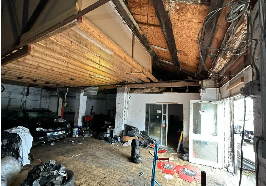
4. Service bay area.
