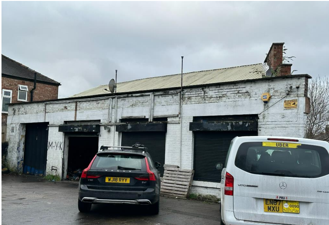
1. Brick built garage/workshop in suburban location.
