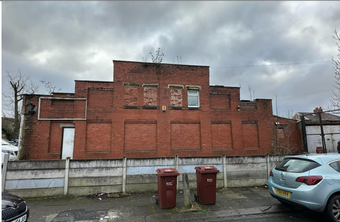
2. Bricked up northern aspect to Monica Grove offering no points of potential ingress.
