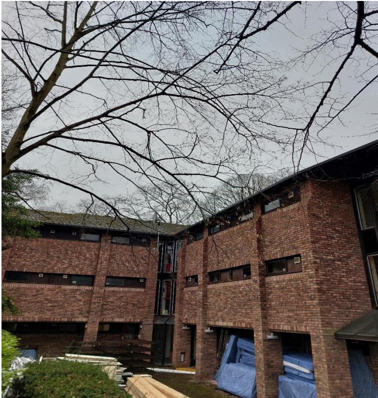
A: Branches overhanging the Plant Room.
