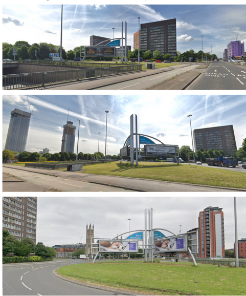
Advertising Structure on the site prior to removal in 2019
