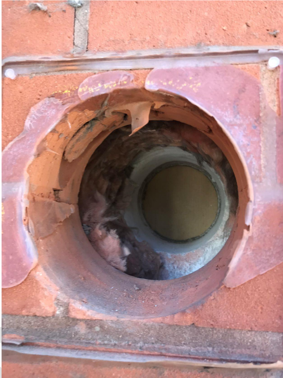
Figure 3 - showing two leaf masonry wall build-up
