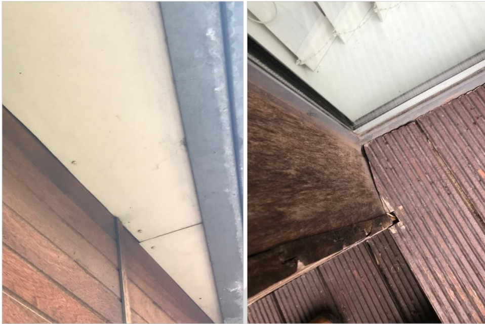
Figure 4 - cladding and soffits around balcony
