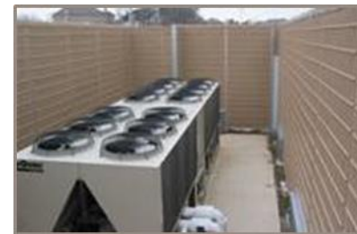
Figure 6—6 Noise barrier with acoustic lining
