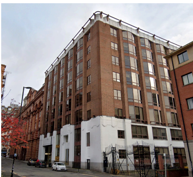
Image 02: Great Bridgewater Street and Lee House side elevations.
