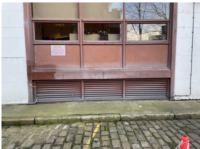
Image 12: View of typical louvre on former Lee House elevation.
