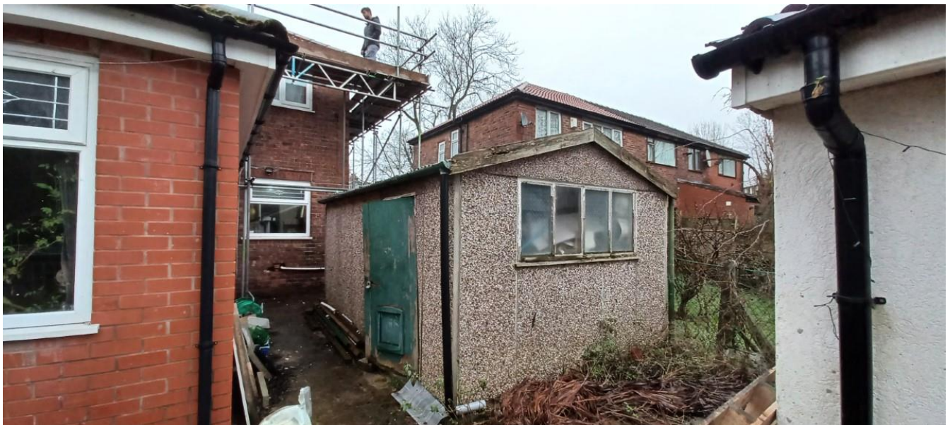
Figure 3. Outbuilding to be removed.
