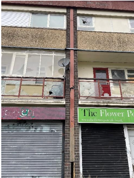
Photograph 8 – Brickwork pillar covered by wooden panel
