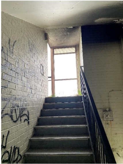
Photograph 3 – Associated stairwell (interior)
