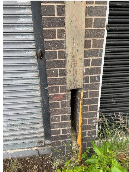
Photograph 9 – Brickwork pillar covered by wooden panel
