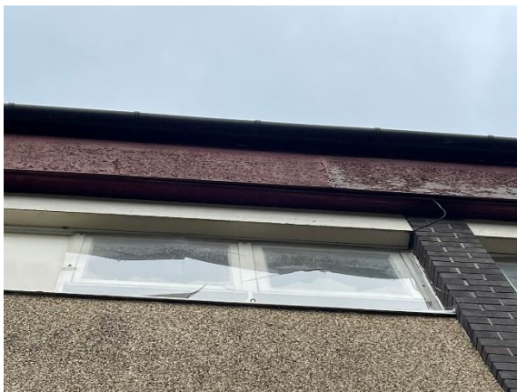
Photograph 7 – Lifting fascia board
