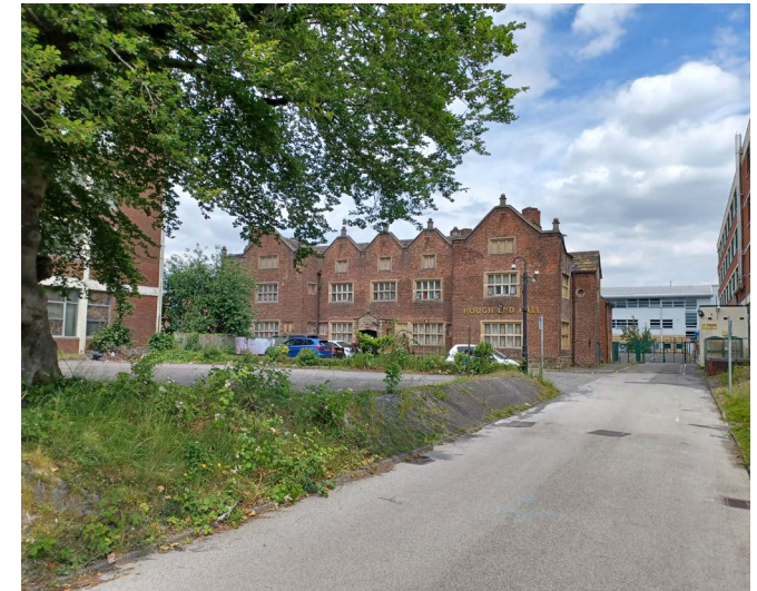
View two - A view of the Hall from the access road
