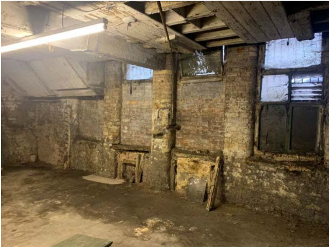
Plate 7 – Basement within 51-53 Richmond Street.
