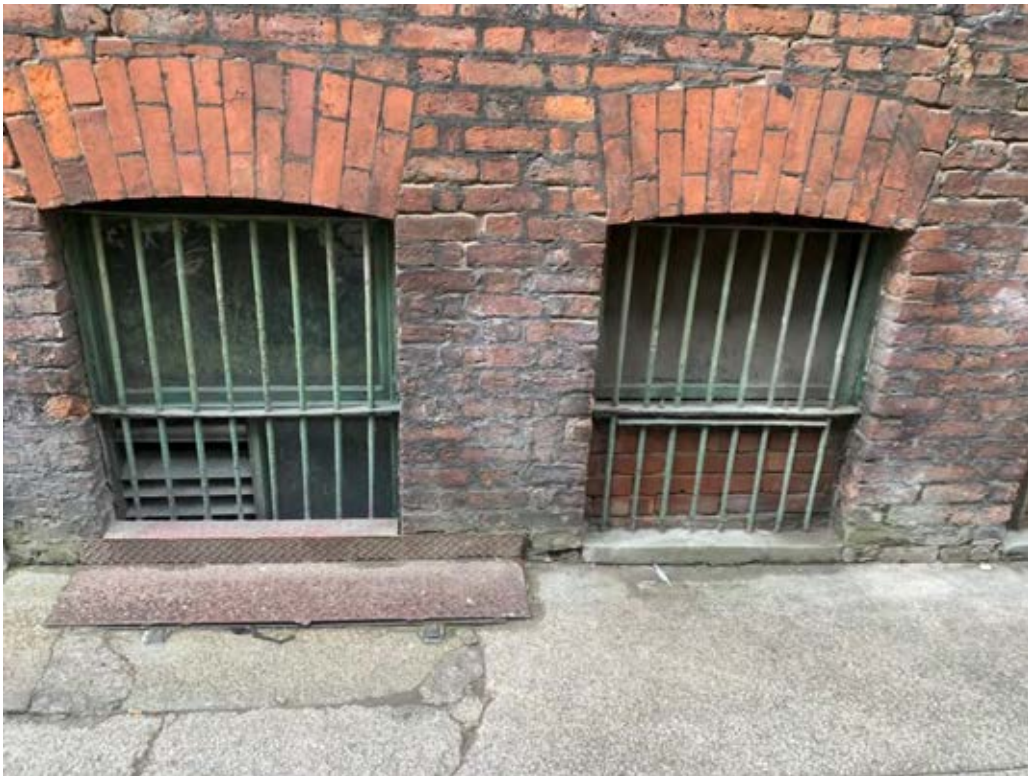
Plate 3 – Basement windows from Richmond Street.
