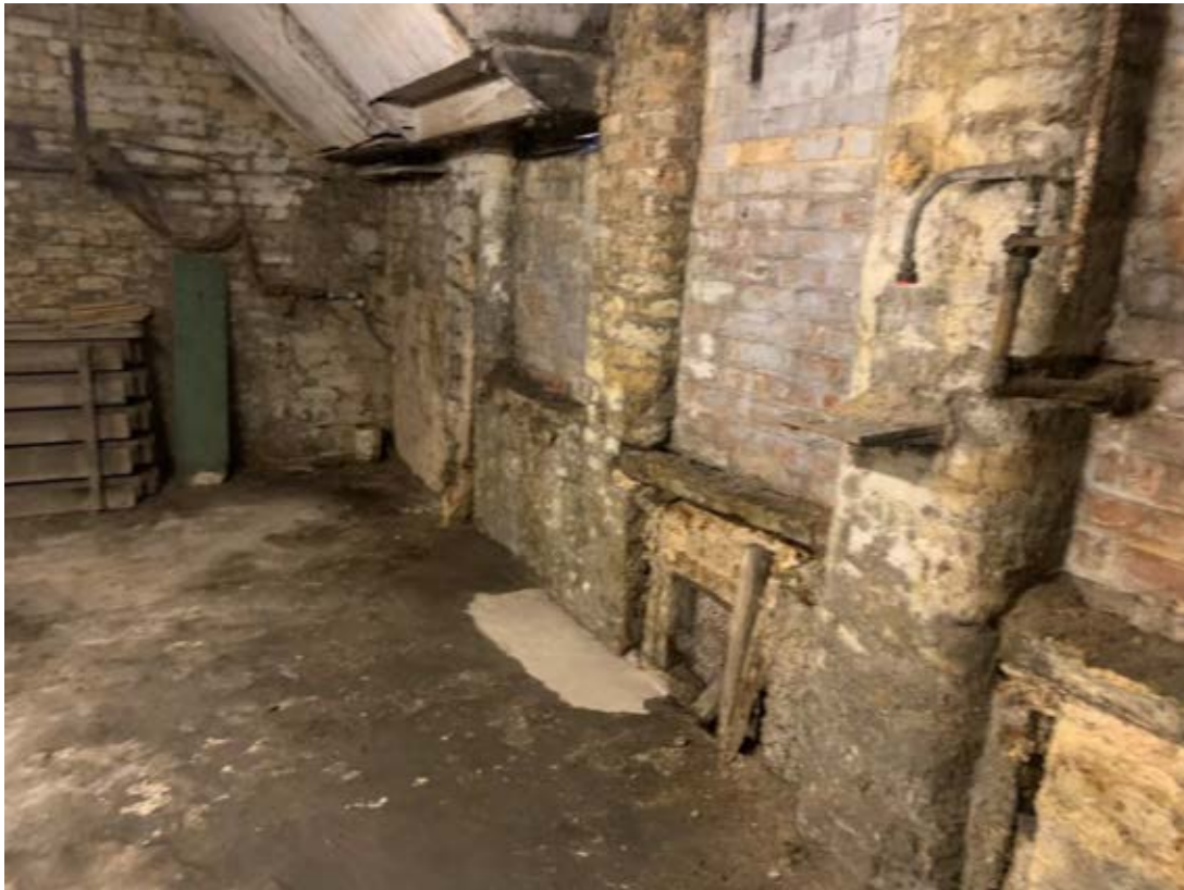
Plate 8 - Basement within 51-53 Richmond Street.
