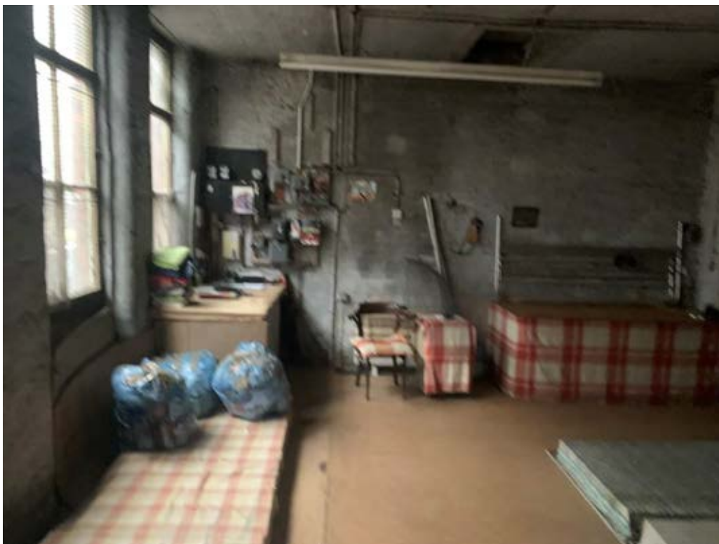
Plate 4 – Ground floor within 51-53 Richmond Street.
