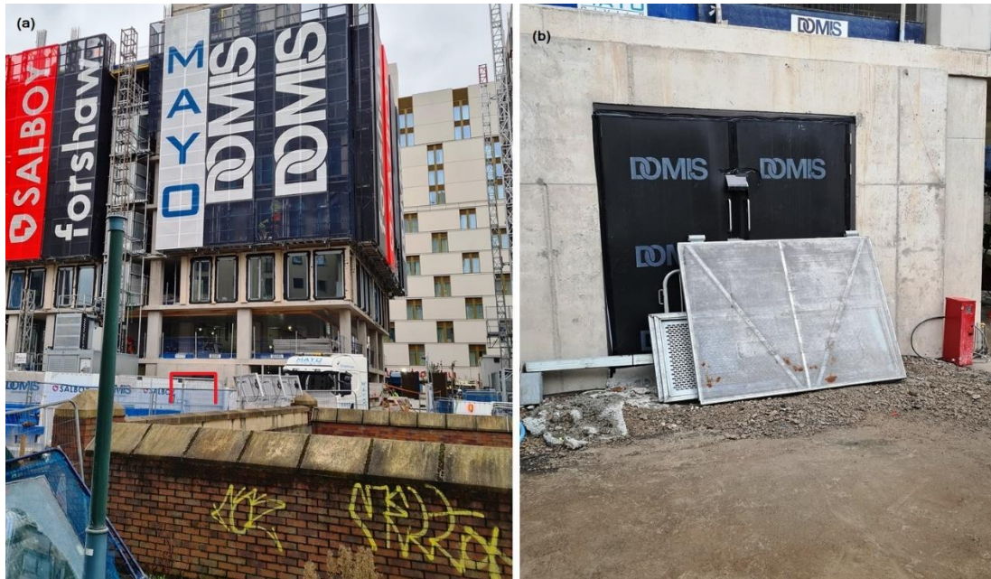
Figure 3.2 Images showing (a) the site with the tram line tunnel (in foreground) and the secondary station on the day of the pre-energisation survey with the substation doors highlighted in red (b) a close up of the substation.
