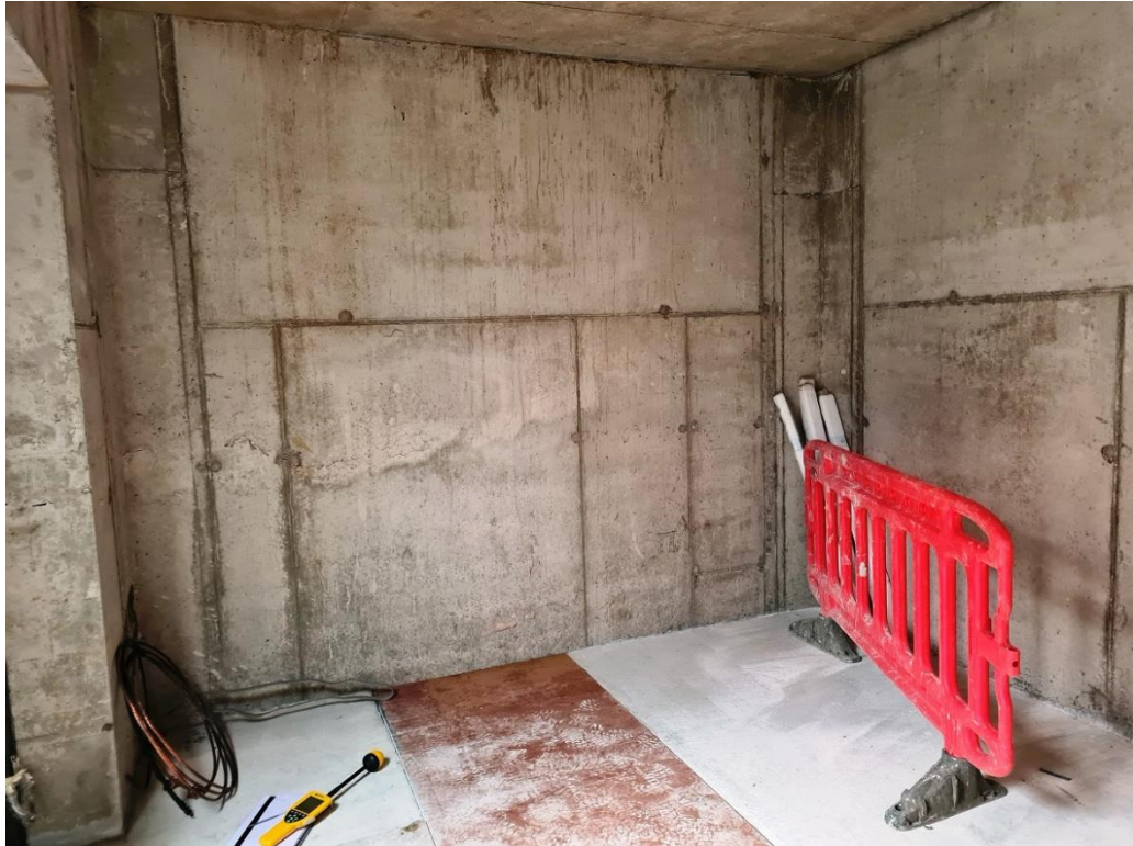
Figure 3.4 Measuring radiofrequency fields at the site within the substation enclosure using the Narda NBM-550.
