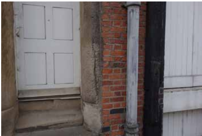
S1038: Spalled bricks. Cut out and replace bricks where erosion exceeds 15mm depth. Repoint using lime mortar.
