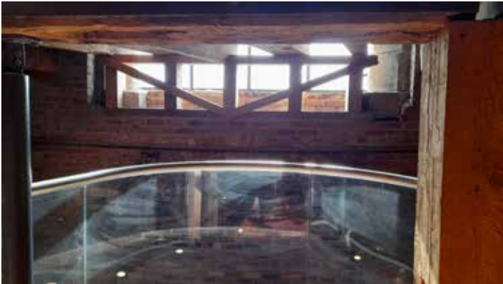
The viaduct level is visible from the landing at ground floor mezzanine
