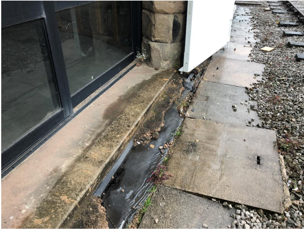
Photograph 15: Bay 5 – detail view of glazing base area
