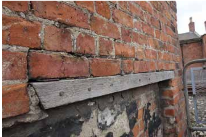
S1076: Corroding emdedded iron duct. Clean and treat where accessible. Repoint around using lime mortar.
