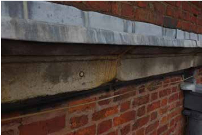
S1007: Bolt shell. Remove bolt shell.
