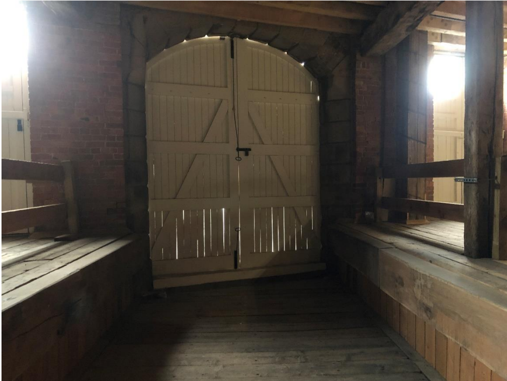
Photograph 10: General internal view at Bay 4 showing locally lowered floor structure to allow goods wagons to enter.
