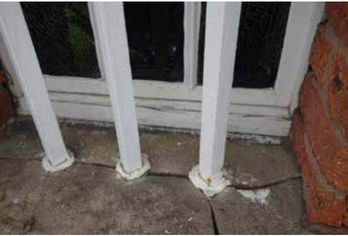
S1006: Corroding metal pipe & material loss to cornice. Remove pipe and undertake indent repair to cornice.
