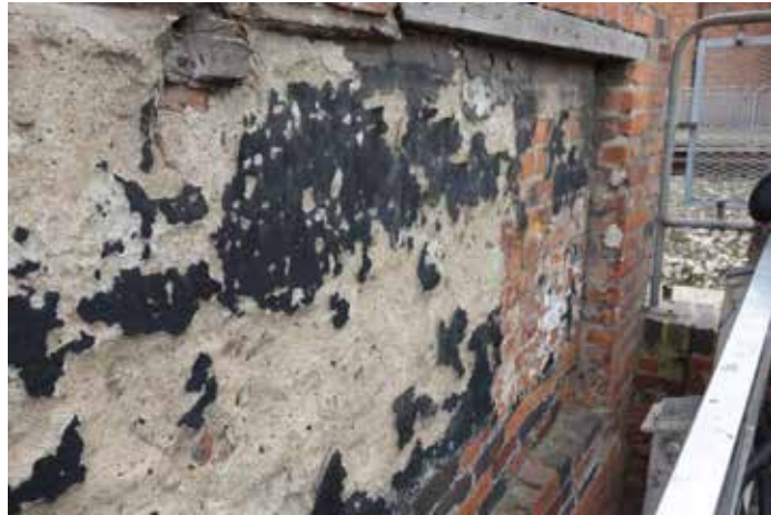
S1075: Multiple vertical cracks in brickwork. Repair using helical bar stitching. Repoint using lime mortar.
