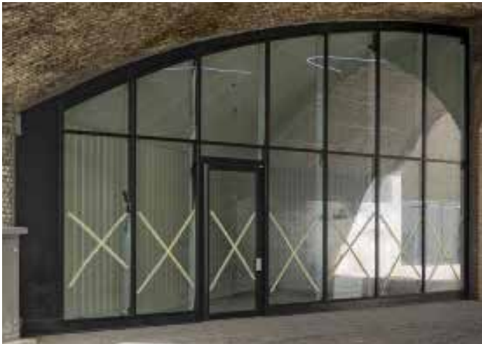
Glazed infill using a glazed infill system with external capping.
