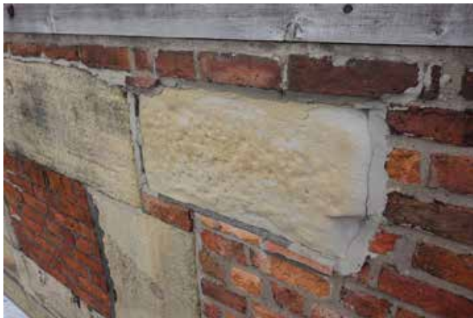
S1065: Delamination of coping blocks (2no.). Indent repair to restore lost section.
