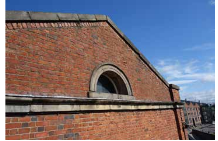
S1028: Delamination at cornice block. Indent repair to stone block.
