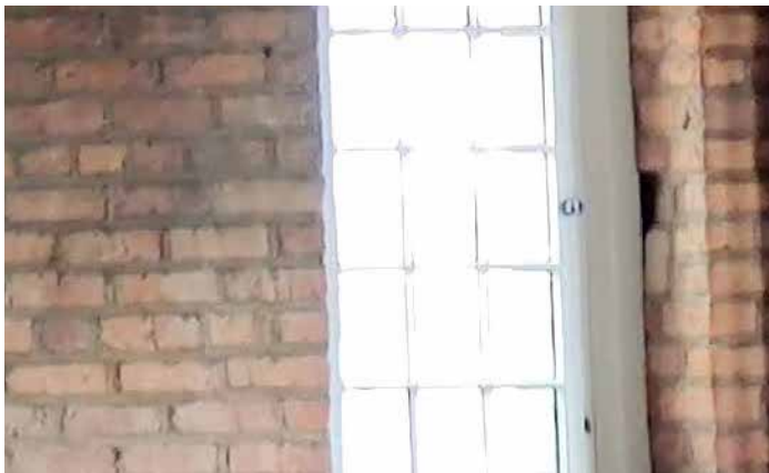
A0046 Brickwork damaged. Brick repair required
