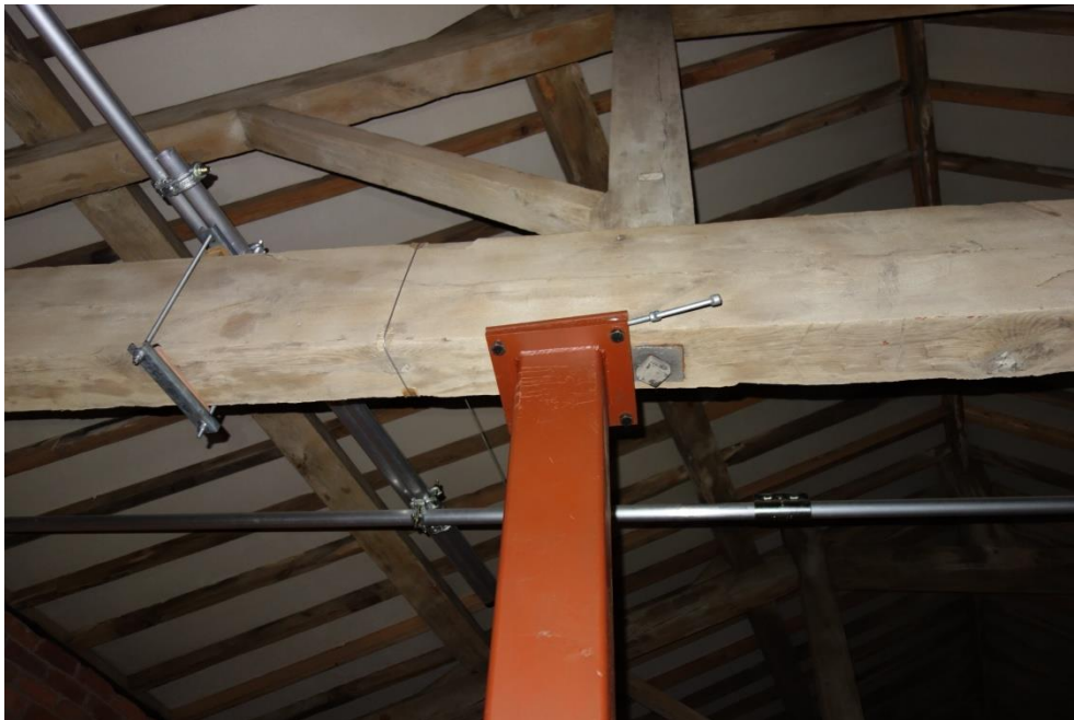
Photograph 22 – The column head plates are pressed firmly to the underside of the trusses using a threaded plate separation system.
