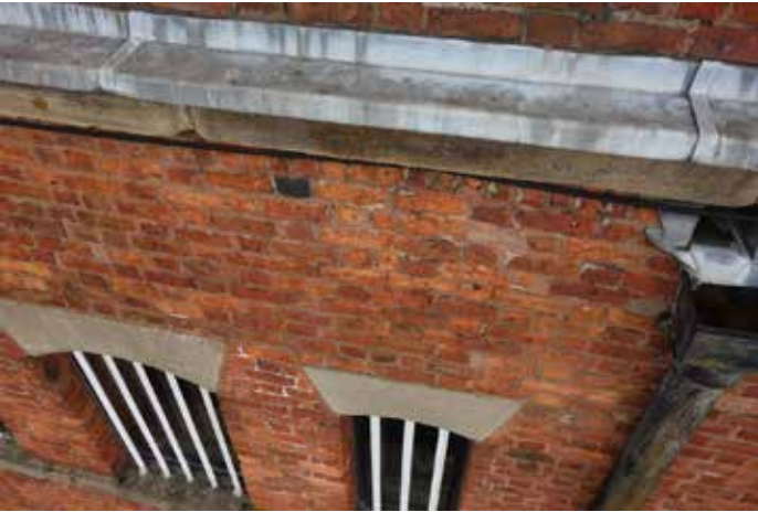
S1002: Spalled bricks. Cut out and replace bricks where erosion exceeds 15mm depth. Repoint using lime mortar.
