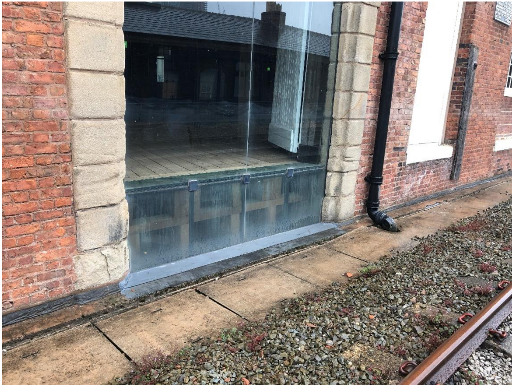
Photograph 8: General external view of glazed opening at Bay 3.
