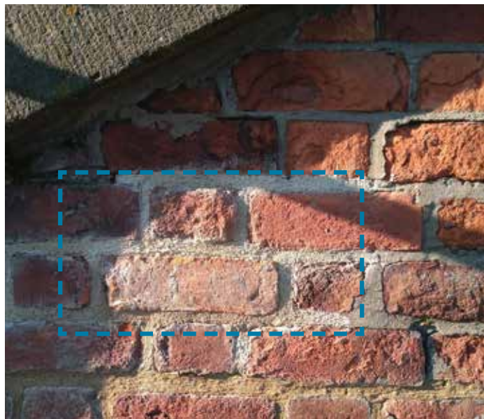
Approved Mortar Sample as CDN/21/0140: Discharge of Condition 4b (samples and specifications of materials) of Listed Building Consent ref:124068/LO/2019
