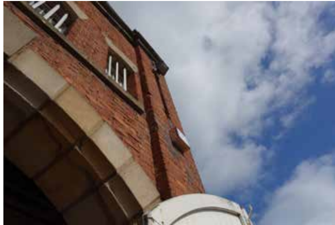
S1030: Spalled bricks. Cut out and replace bricks where erosion exceeds 15mm depth. Repoint using lime mortar.
