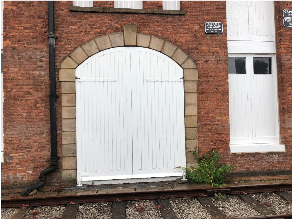
Photograph 11: General external view showing timber door and sill.
