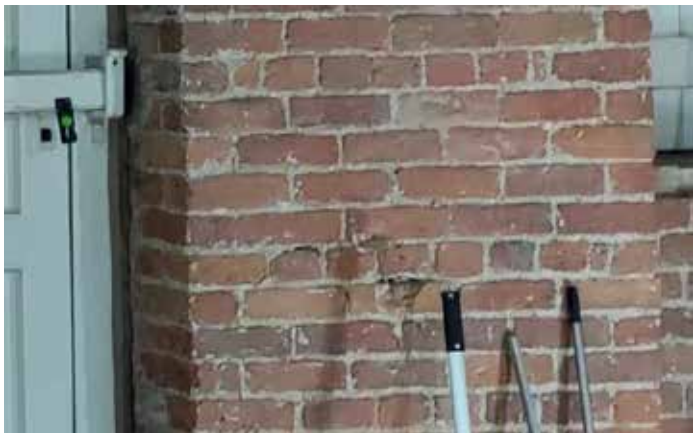
A0038: Brickwork damaged. Brick repair required
