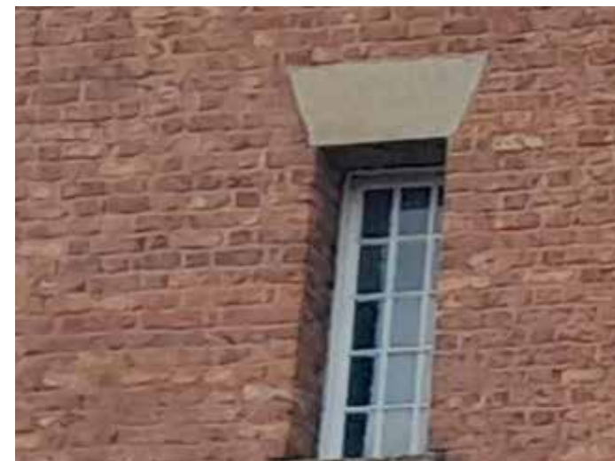
A1023: East elevation frames to be redecorated.
