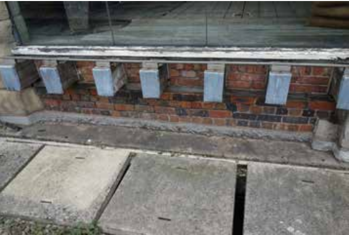
S1005: 7no. Decayed timber joists below glazed opening. Replace with new timber to match.
