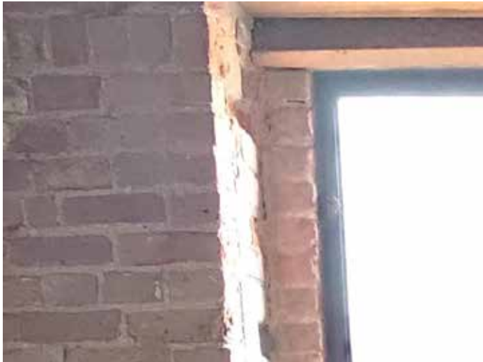
A0038: Brickwork damaged. Brick repair required
