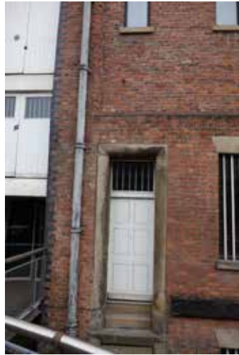
S1050: Open joints to stone architrave blocks. Repoint using lime mortar.
