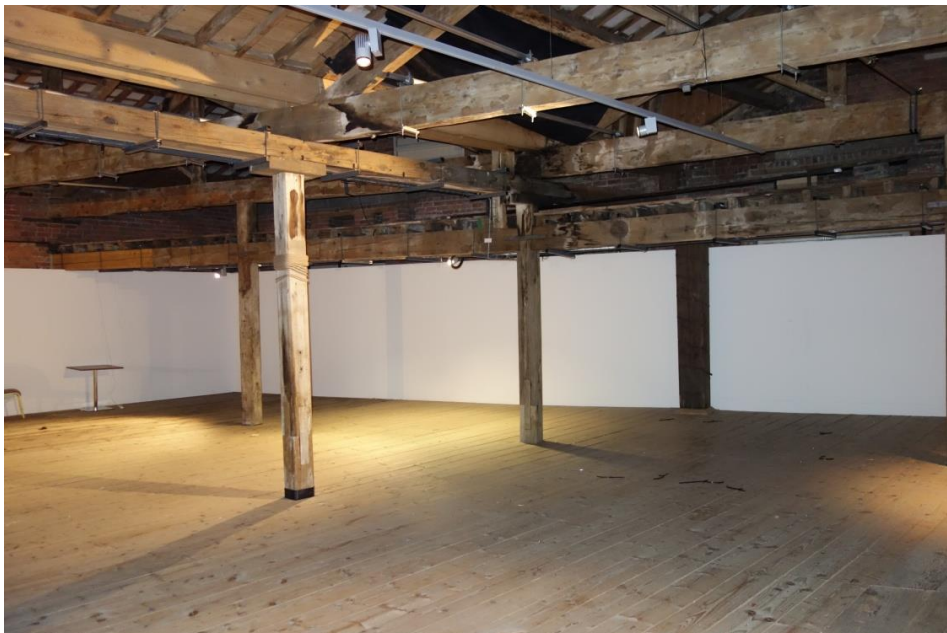
Photograph 20 – A general view of the top floor of the building, showing typical arrangement of regularly spaced timber columns, block corbel heads and primary valley beams onto which the timber Queen post trusses sit.
