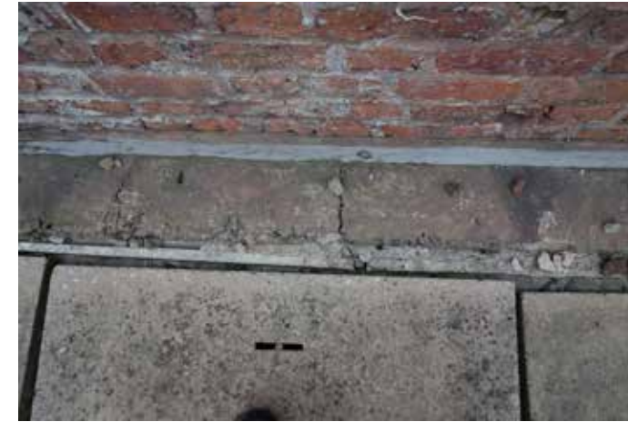
S1015: Crack through drainage channel at wall base. Further investigation required as part of viaduct drainage strategy.
