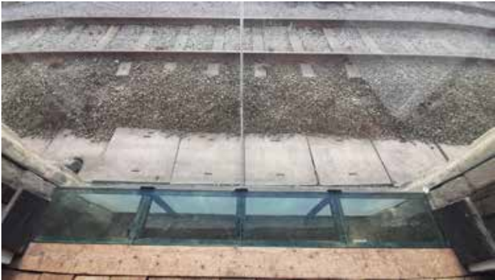
As with Bay 1, Bay has a glass floor with structure bearing down on a timber batten
