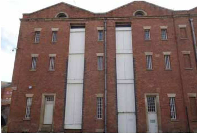
S1038: Spalled bricks. Cut out and replace bricks where erosion exceeds 15mm depth. Repoint using lime mortar.
