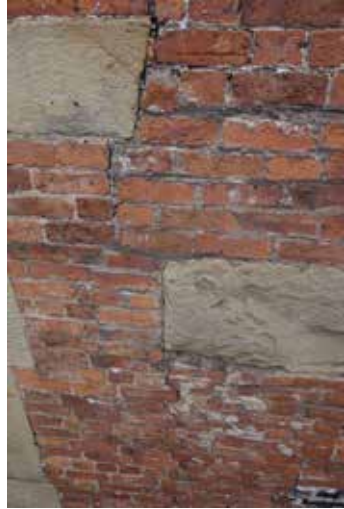
S1075: Multiple vertical cracks in brickwork. Repair using helical bar stitching. Repoint using lime mortar.
