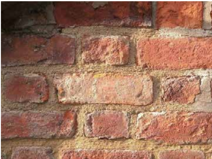
Salvaged brick from client stocks on site. The replacement brick has been set out and aligned carefully to ensure interfaces and junctions with existing masonry is maintained. Joint widths have been maintained and replicated. The salvaged brick has been laid will be laid and sighted on a full bed of mortar with all joints filled.
