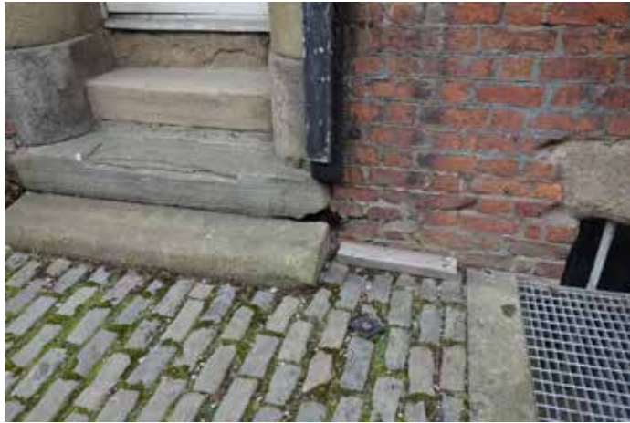
S1061: Spalled and eroded step treads. Indent repairs to 2no. treads.
