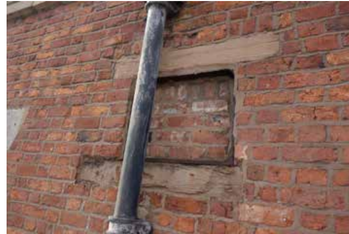
S1031: Metal duct frame is corroded. Cut out and brick in the opening.
