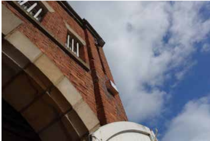
S1029: Material loss/spall. Indent repair to stone block.
