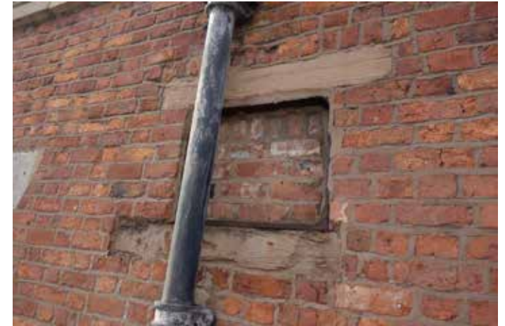
S1028: Delamination at cornice block. Indent repair to stone block.
