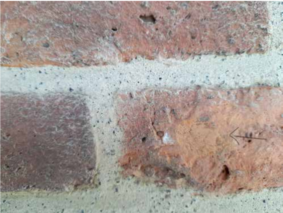
Brickdust repair to Cemtie
