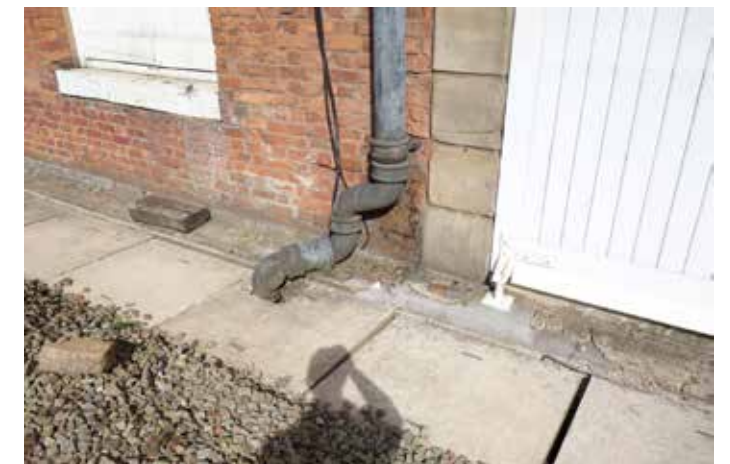
S1020: Patches of eroded pointing. Repoint using lime mortar.
