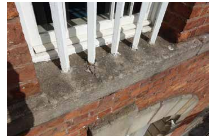
S1020: Patches of eroded pointing. Repoint using lime mortar.
