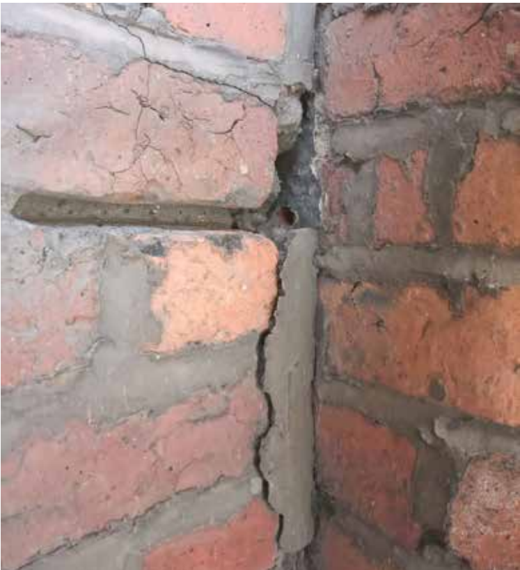
Helifix chase cut to corner
