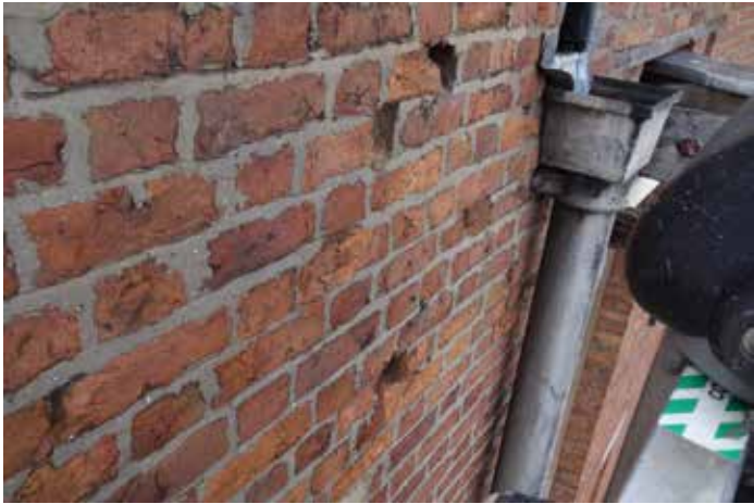
S1040: Spalled bricks. Cut out and replace bricks where erosion exceeds 15mm depth. Repoint using lime mortar.
