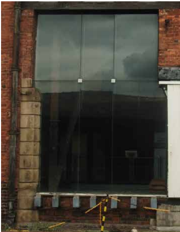
Bay 2 wagon arch was adapted in 1870 as a result of technological change,
