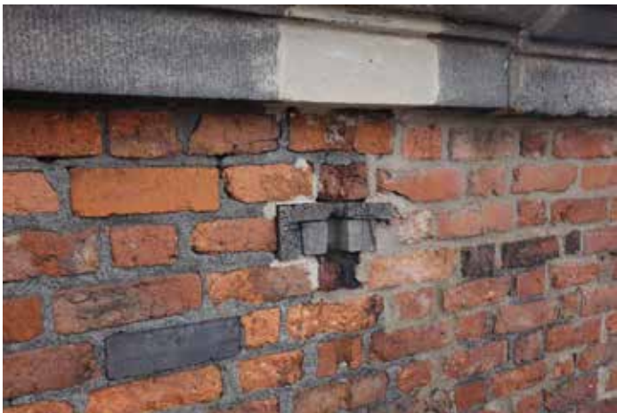
S1064: Delamination of LHS pediment block face. Indent repair to restore lost section.
