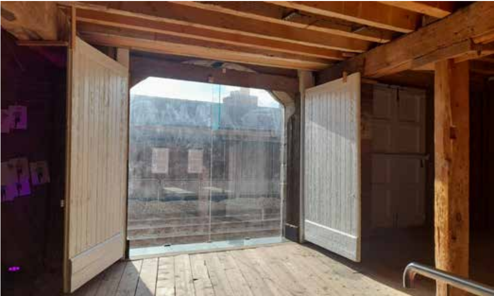
View out of Bay 3, which is a point of arrival from the steps from the lower yard entrance
