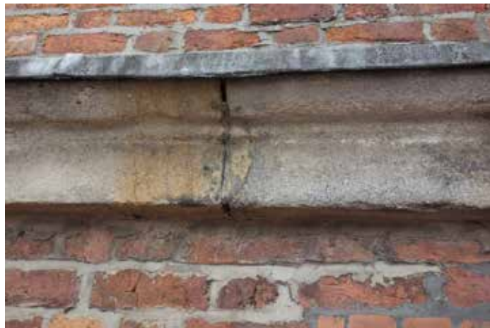
S1054: Patches of eroded pointing. Repoint using lime mortar.
