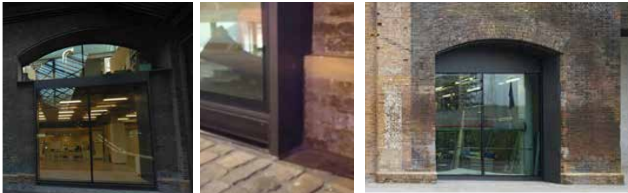
Infill of glazing to former railway goods buildings in King's Cross. The abutting frame extends forward of the brickwork. The glazing element is simple and the transom defined.
