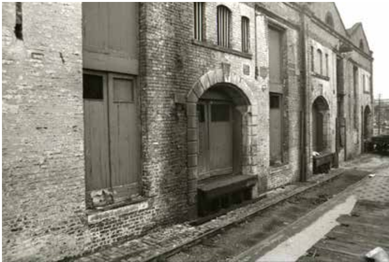
Close-up view of the Bay 4 wagon arch (centre) and Bay 5 wagon arches to the right of the picture. Undated photograph pre-museum occupation. Source: unknown.
