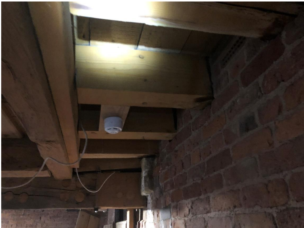
Photograph 6: Internal view showing the timber framing arrangement and joists passing through the wall.
