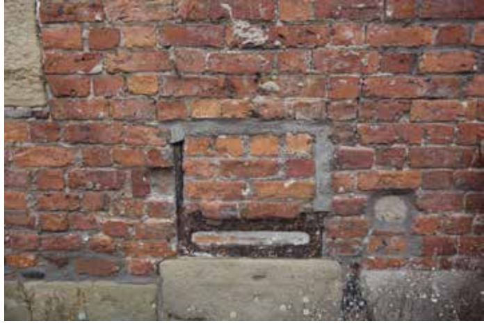
S1076: Corroding emdedded iron duct. Clean and treat where accessible. Repoint around using lime mortar.
