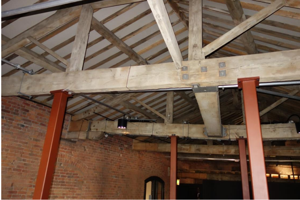
Photograph 21 – Square Hollow Section columns (4No), serve to prop failed trusses at the East side of Bay 2.
