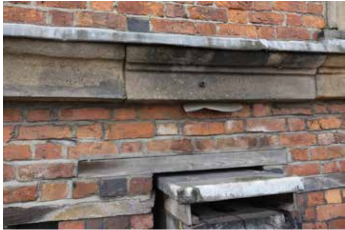
S1052: Bolt shells in cornice blocks. Remove and infill holes using lime mortar.
