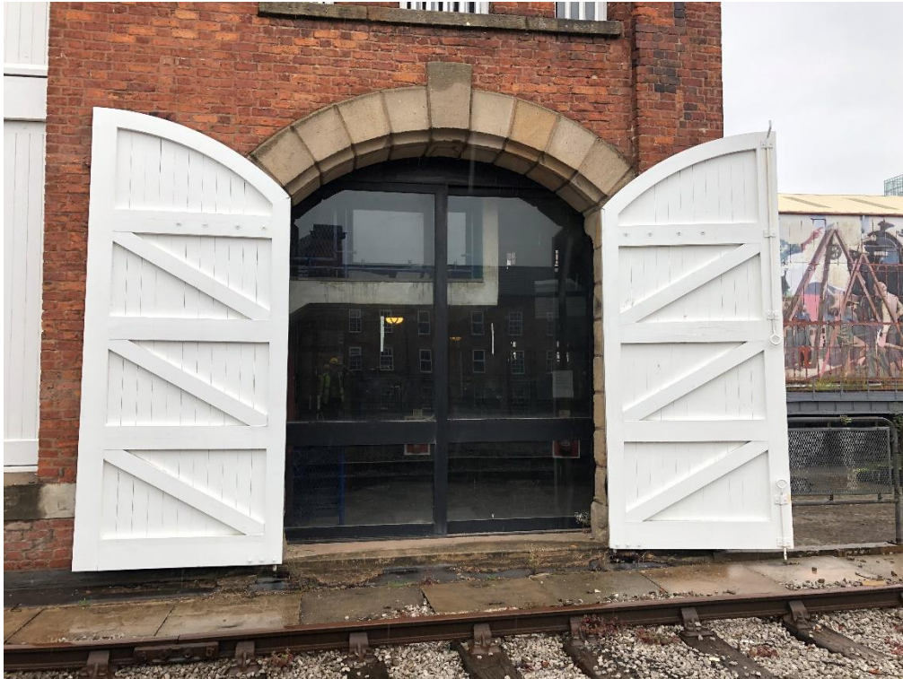
Photograph 14: Bay 5 – left-hand (west) door opening.
