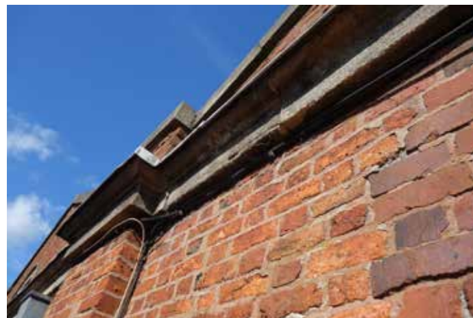
S1018: Material loss/spall. Indent repair to stone block.
