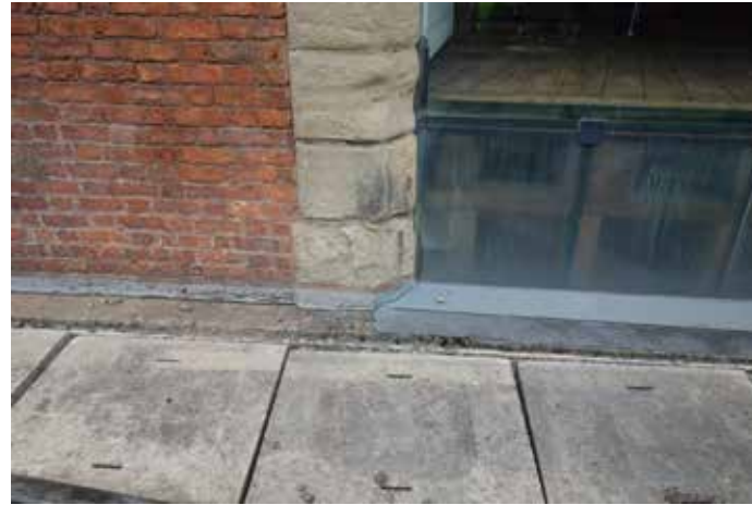
S1014: Material loss/spall. Indent repair to stone block.
