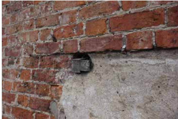
S1074: Previous surface repair failing. Indent repair to restore lost section.
