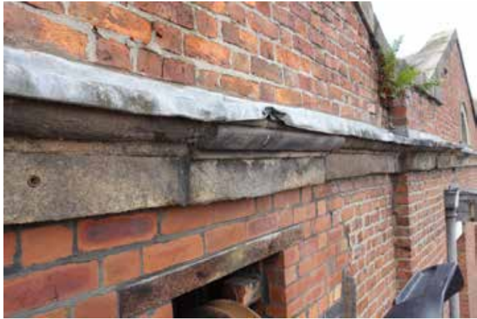
S1049: Bolt shells in cornice blocks. Remove and infill holes using lime mortar.
