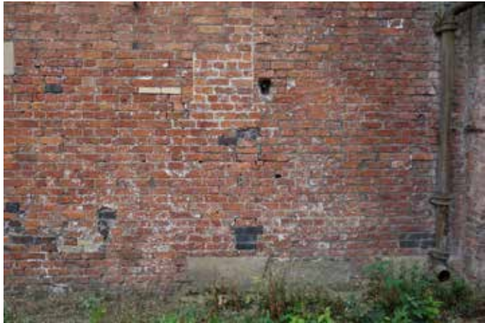
S1073: Multiple vertical cracks in brickwork. Repair using helical bar stitching. Repoint using lime mortar.
