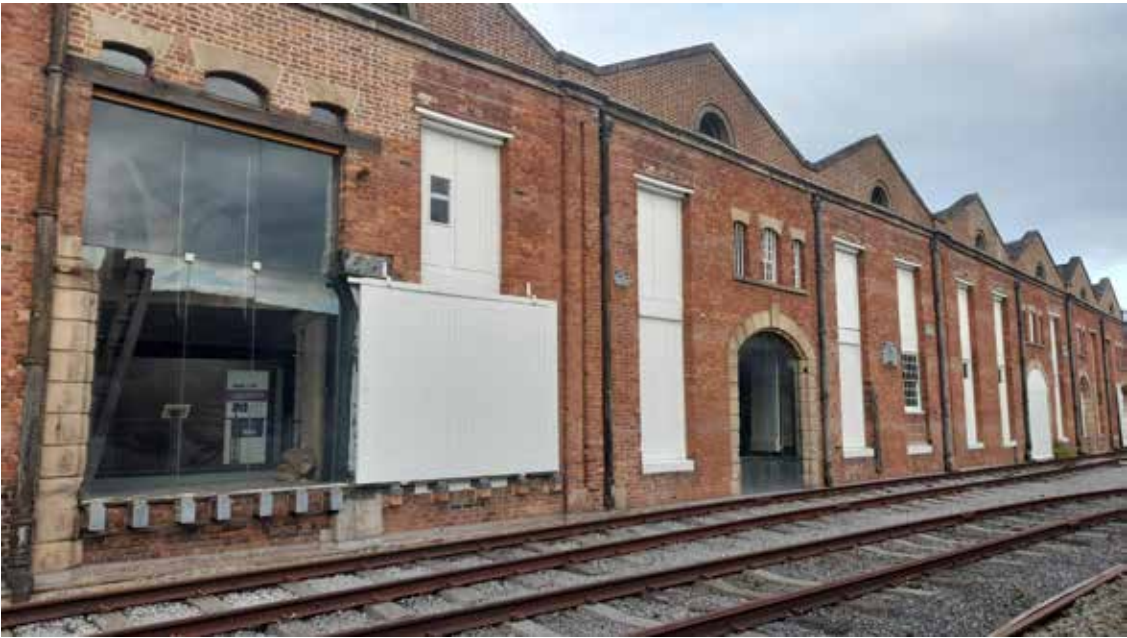
Bay 2 foreground, and Bay 3 to the right. The Bay 3 detail to the viaduct is the same as Bay 1
