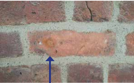
Example of hole repair to brick after removal of redundant fixing, Filled with brick dust and mortar mix to blend with adjacent brick colour.
