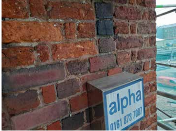
A1043: Modern brickwork. Replaced with salvaged brick
