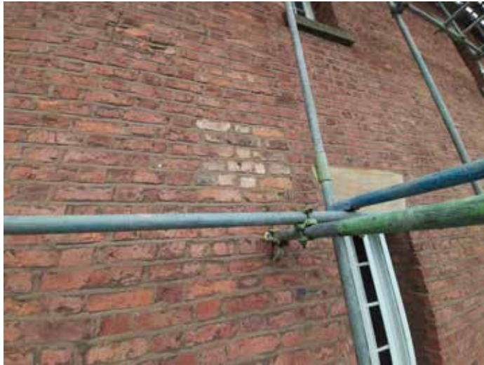
A1025: Modern brickwork. Replace with salvaged brick
