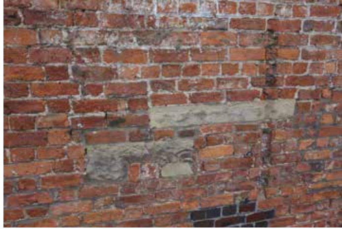
S1074: Previous surface repair failing. Indent repair to restore lost section.
