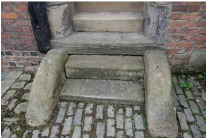
S1051: Settlement of steps. Dismantle and rebuild on new foundation.
