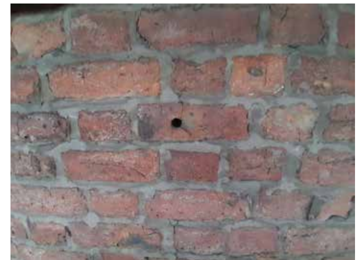
A1024: Hole in brickwall. Brick repairs correctly with brick dust
