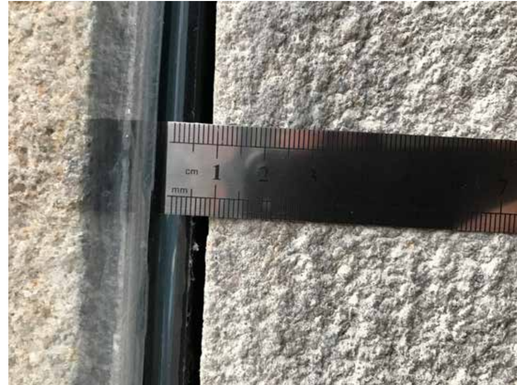
View of existing detail at Bay 3.
