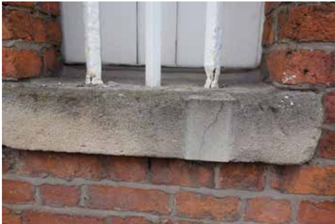
S1042: Vertical crack/fissure in stone architrave. Pin fissure using stainless steel dowels, Infill with colour matched repair mortar.
