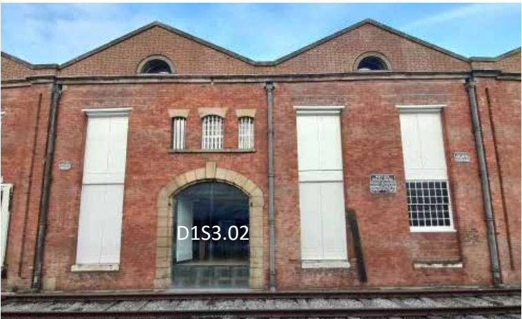
Wagon Arch D1S3.02 Externally: • Single layer of structural glazing, glass fins • Glazing extends to the level of trackbed. • Timber Cargo door behind • Arched opening of stonework •
