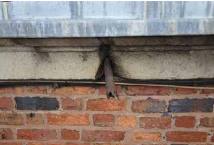
S1002: Spalled bricks. Cut out and replace bricks where erosion exceeds 15mm depth. Repoint using lime mortar.
