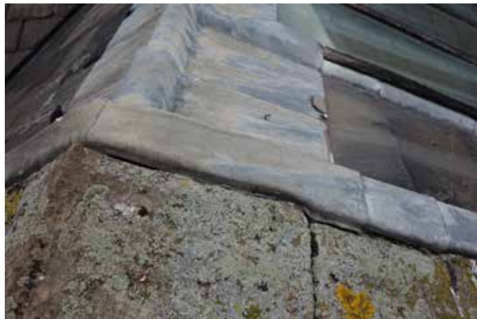
S1062: Corroding metal pin. Remove pin and repoint crack using lime mortar.
