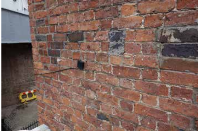
S1073: Multiple vertical cracks in brickwork. Repair using helical bar stitching. Repoint using lime mortar.
