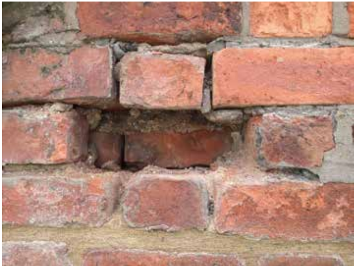
Failed brick removed. Remaining adjacent masonry is not disturbed, marked or damaged during this process. All joint surfaces to be left in a suitable condition to receive the replacement brick.
