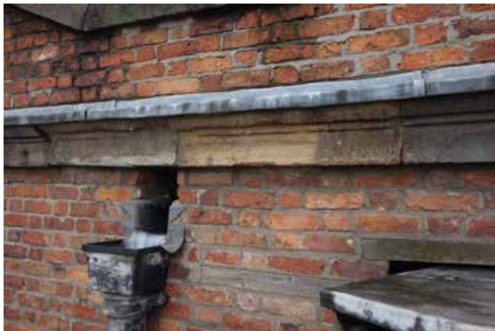
S1053: Spalled bricks. Cut out and replace bricks where erosion exceeds 15mm depth. Repoint using lime mortar.
