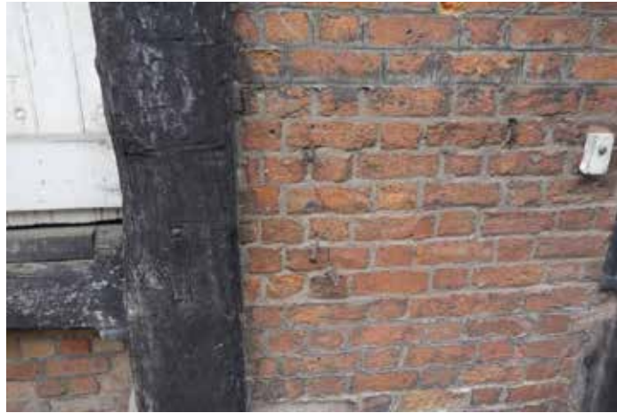
S1062: Corroding metal pin. Remove pin and repoint crack using lime mortar.
