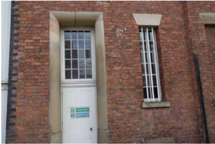
S1039: Previously repaired crack to door head, c6mm width. Rake out cementitious mortar, repoint with lime mortar.
