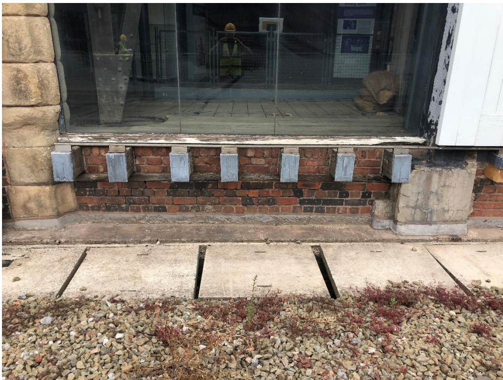
Photograph 4: General external view of the base of the glazing showing floor joists projecting through the wall.
