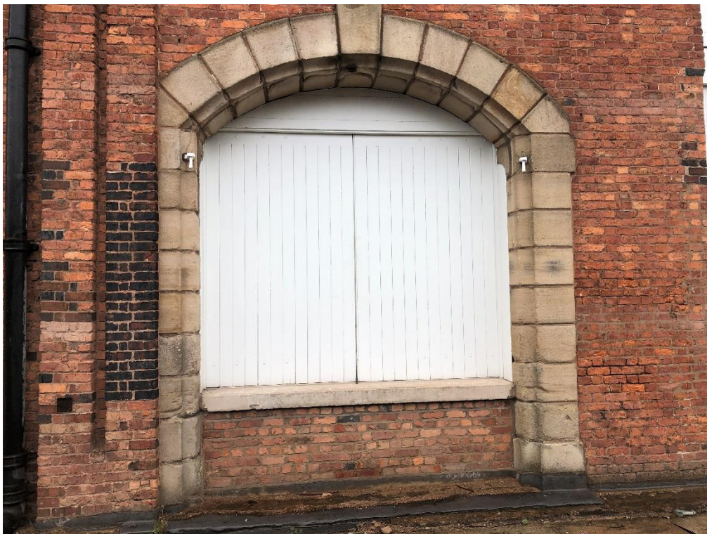
Photograph 13: Bay 5 – left-hand (west) door opening.
