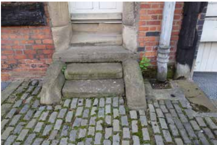
S1040: Spalled bricks. Cut out and replace bricks where erosion exceeds 15mm depth. Repoint using lime mortar.
