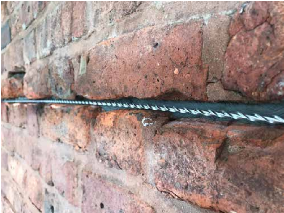
Helibar inserted
