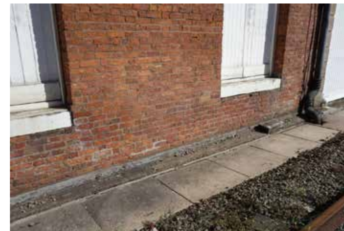
S1015: Crack through drainage channel at wall base. Further investigation required as part of viaduct drainage strategy.
