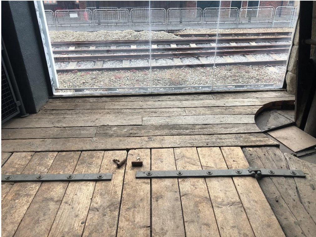
Photograph 5: General internal view of the glazed opening.
