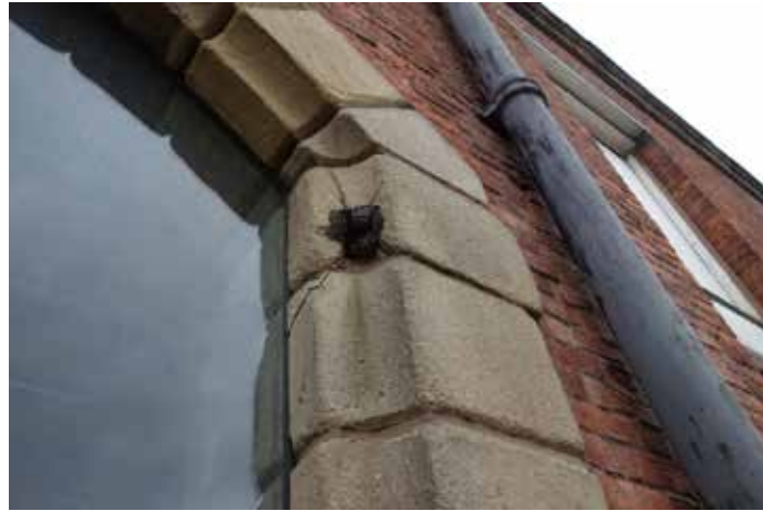
S1013: Crack/spall to block at hinge fixing. Treat ironwork, indent repair to stone block.
