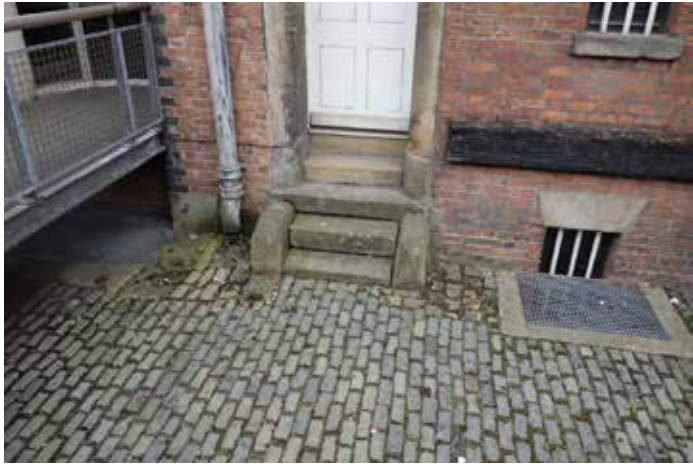
S1051: Settlement of steps. Dismantle and rebuild on new foundation.
