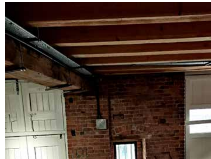
A0068: Wood blocks inserted to wall. Remove and replaced with salvaged bricks
