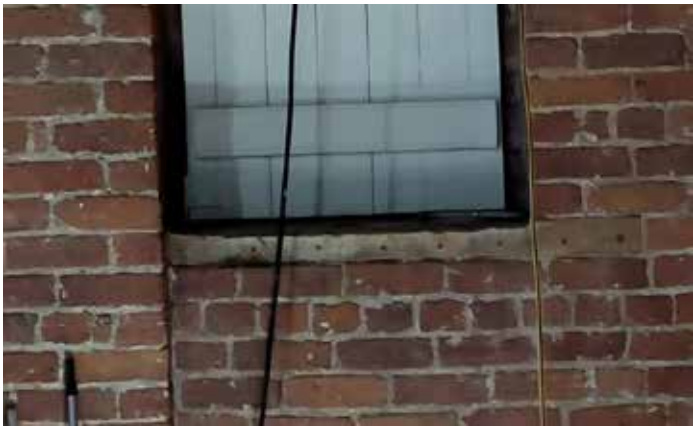
A0040: Poor pointing. Brick repair required
