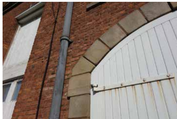
S1018: Material loss/spall. Indent repair to stone block.
