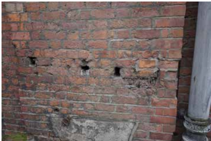
S1049: Bolt shells in cornice blocks. Remove and infill holes using lime mortar.
