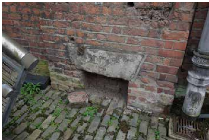
S1050: Open joints to stone architrave blocks. Repoint using lime mortar.
