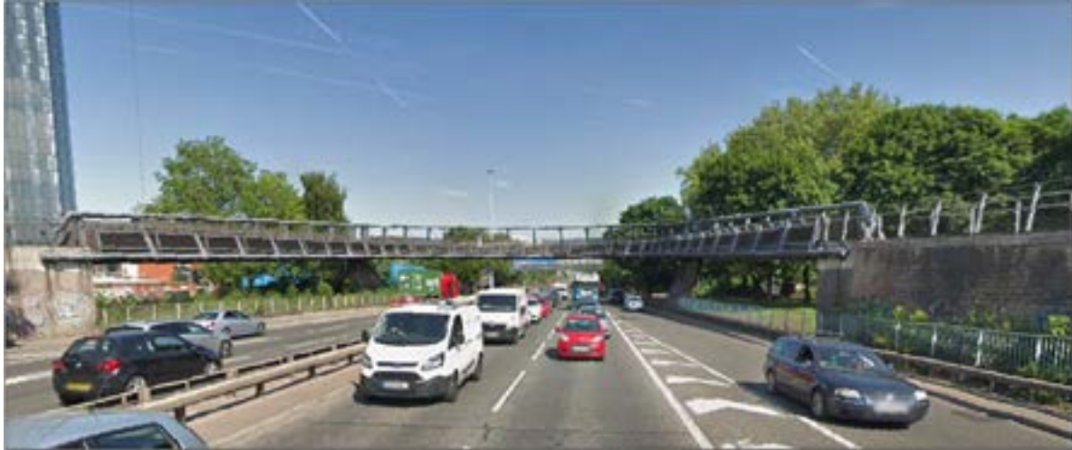
Figure 5.1: Footbridge over the A57 Mancunian Way
