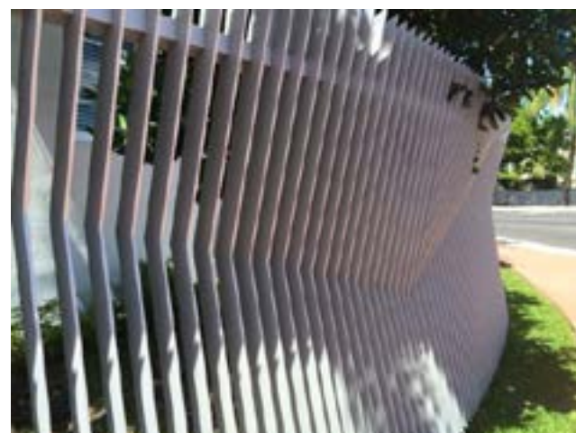
Rear RHS rail supporting the aluminium fence
