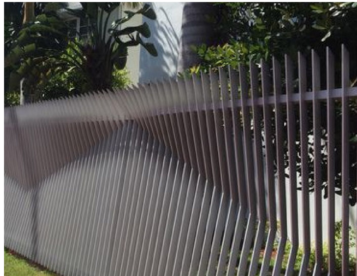
RHS rail supporting the aluminium fence
