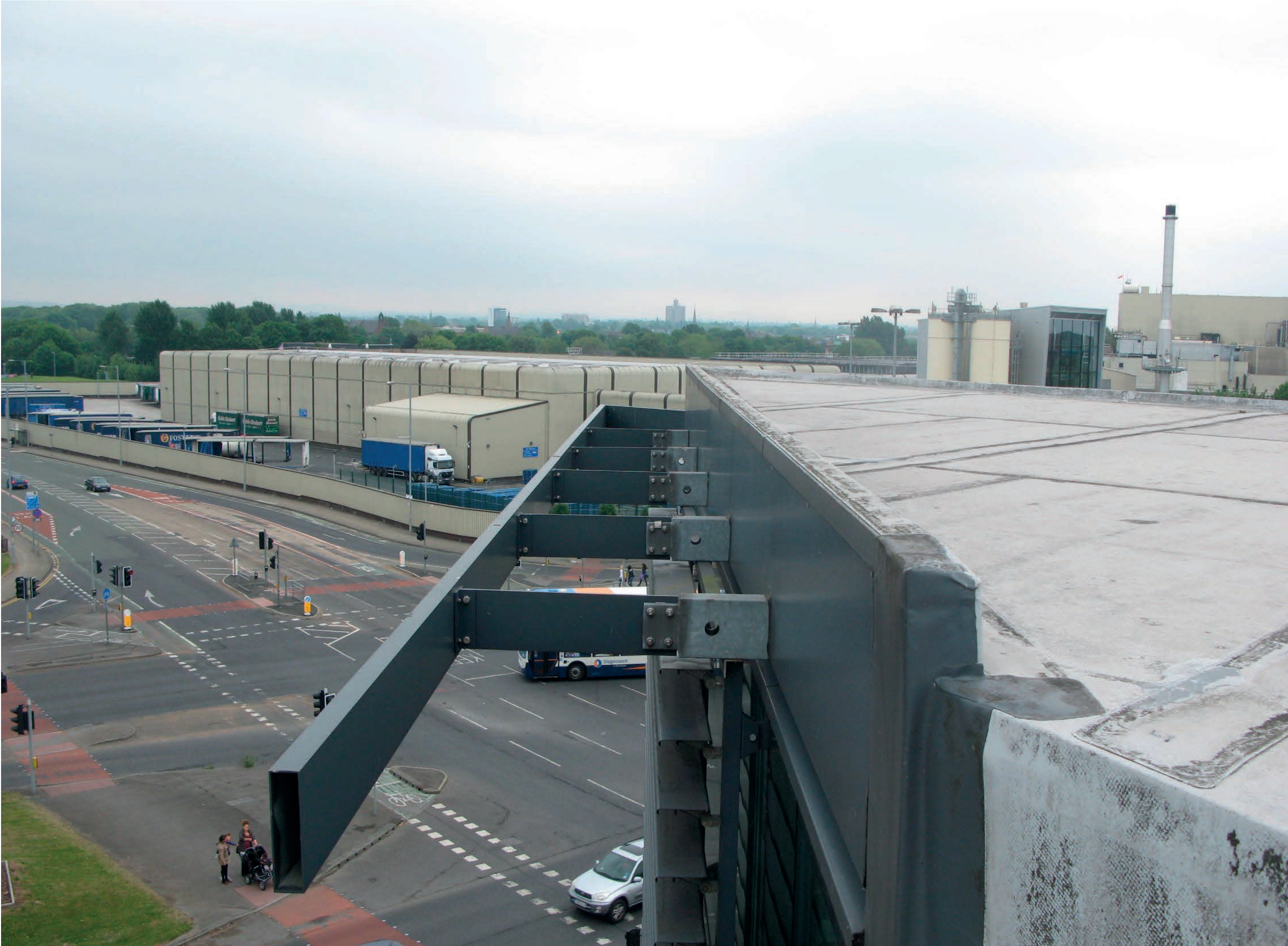
IMAGES SHOWING EXISTING BRACKETS FOR FIXING IN TO
