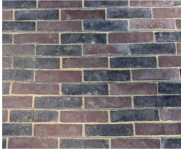
SAMPLE PANEL REVIEWED ON SITE
